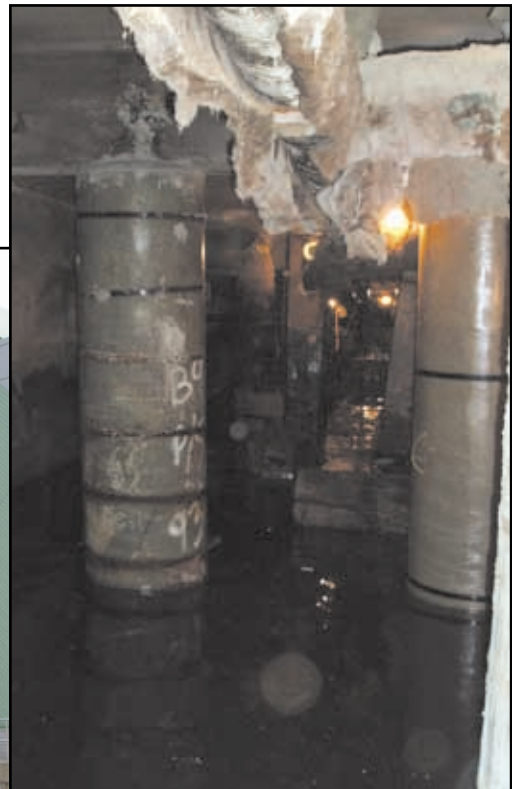
Above: Completed Fiber-Form installation to the timber piles.
