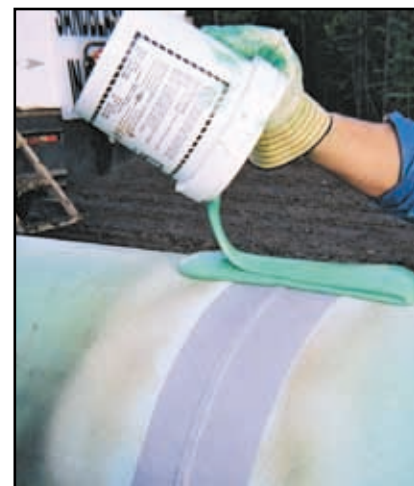
Denso Protal 7200 is applied above the weld area of the pipe, prior to being spread out over it with a hand roller.
