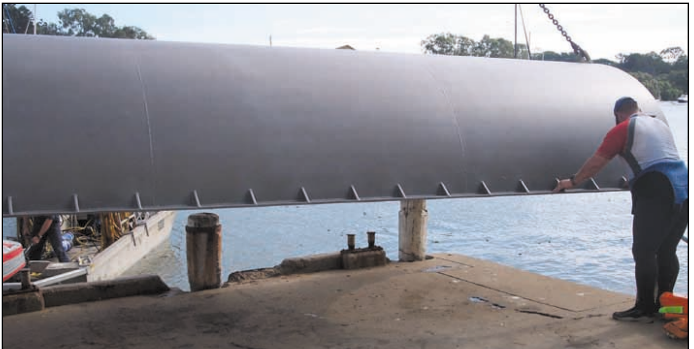
Below: The steel sleeve coated with Denso Rigspray Micro being lifted from a nearby pier.
