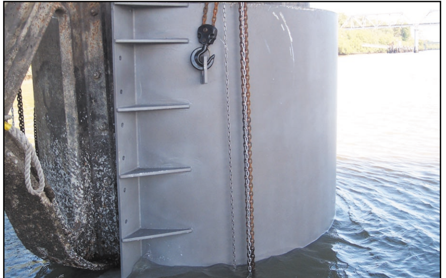
Above: The sleeve being fixed into position around the damaged bridge pylon.
