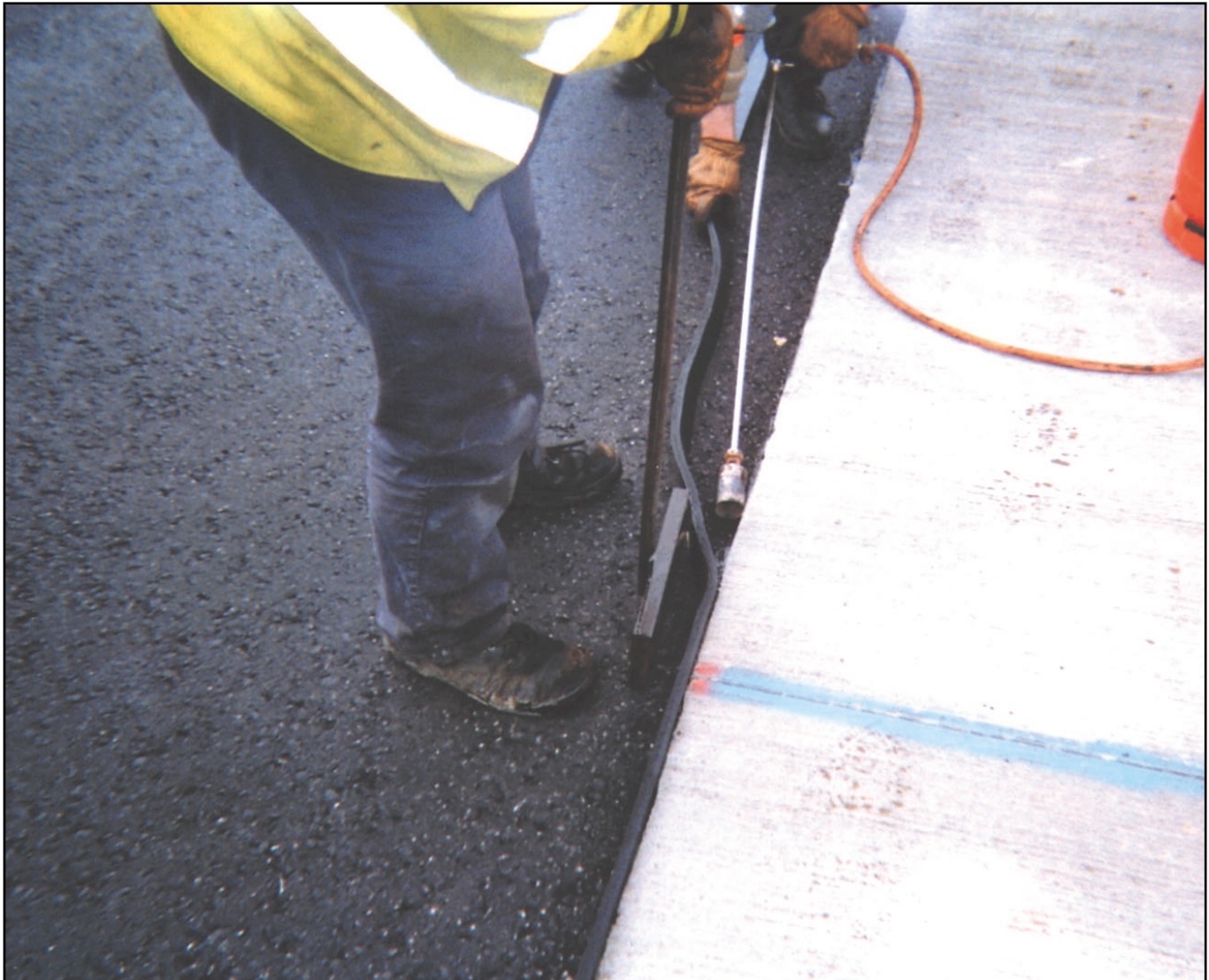
The application of Densoband to the joint face of the new concrete aircraft servicing platform at RAF Waddington.
