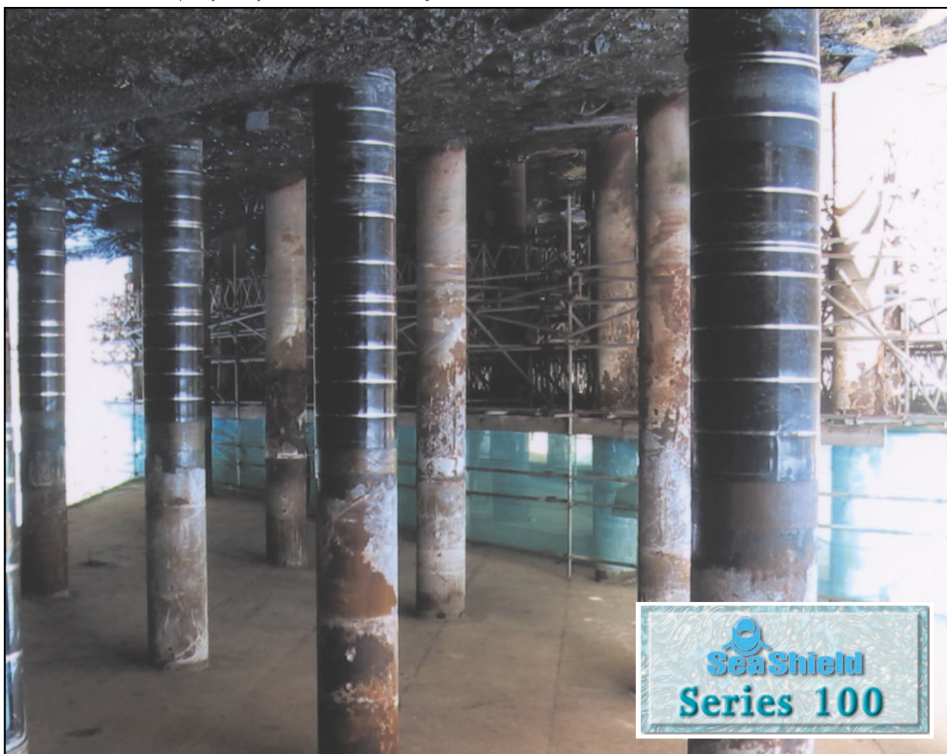
View of the SeaShield Series 100 System protected piles under the Hadrian Road Bridge.
