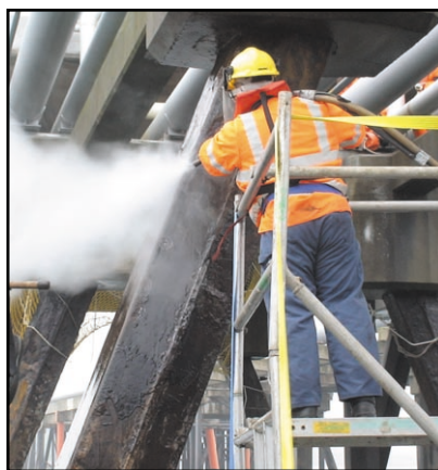
Above: Water jetting in progress.
