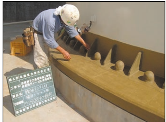
Densyl Tape and Denso Hi-Tack Tape completes the ultra-conformable protective system.
