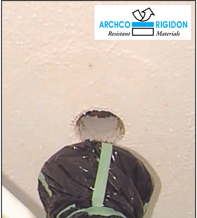
The finished Archco 432D lining.
