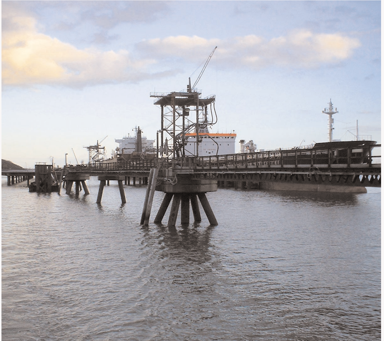
Milford Haven terminal, jetty piles protected with SeaShield 2000HD - See story page 11.
