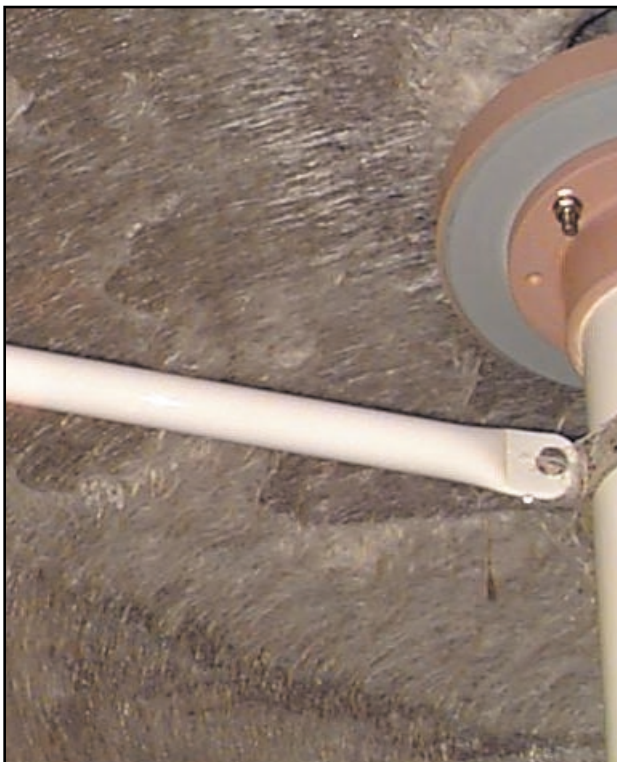
Before the application of the lining.
