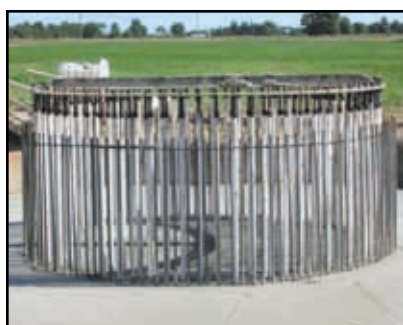
Re-bar rods being installed on site.
