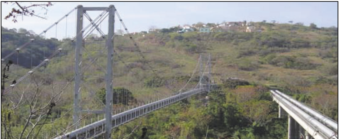
Durban Metro pipe bridge - Denso Steelcoat Systems have been in use in South Africa since 1978
