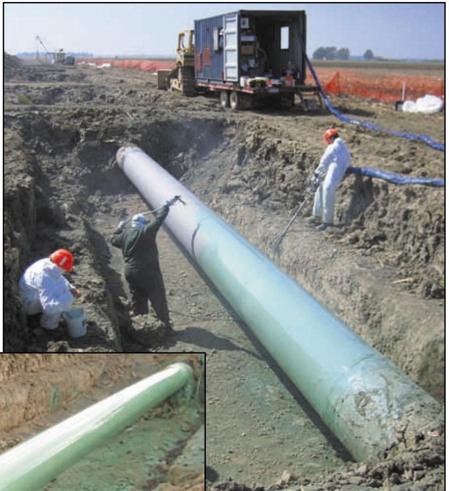
Top: Removal of old coal tar enamel coating.
