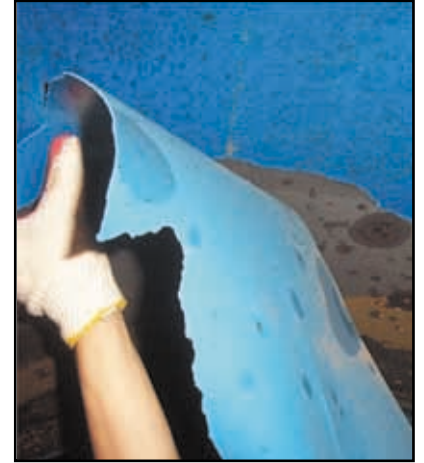
Above: The original lining has reached the end of its life.
