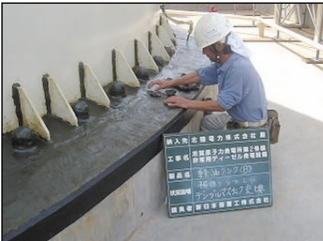
Densyl Mastic is used to create a smooth profile around any irregular shapes.
