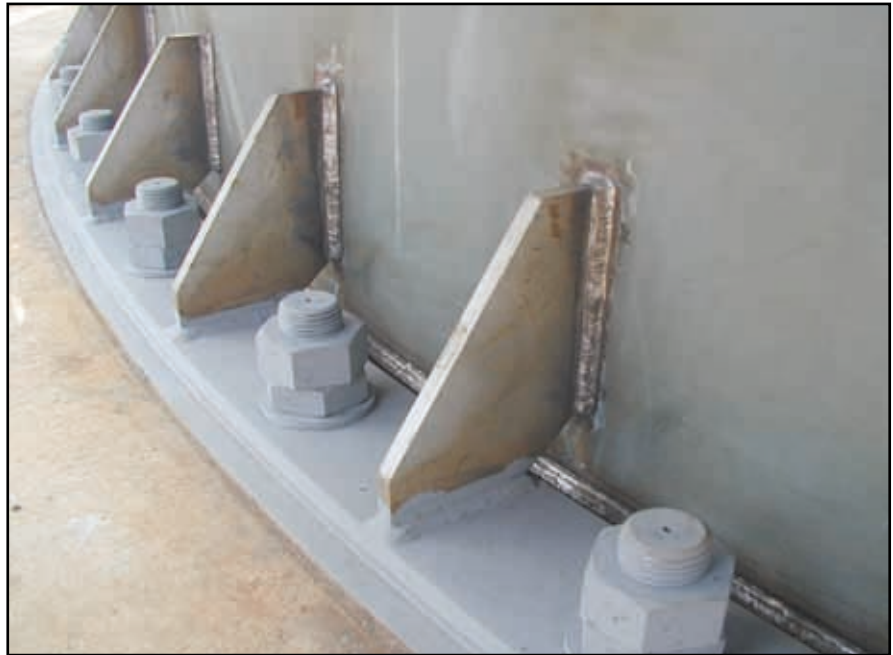
The tank base cleaned and ready for the application of the Denso system.
