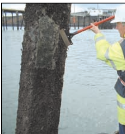
Above: Initial cleaning underway prior to water jetting.
