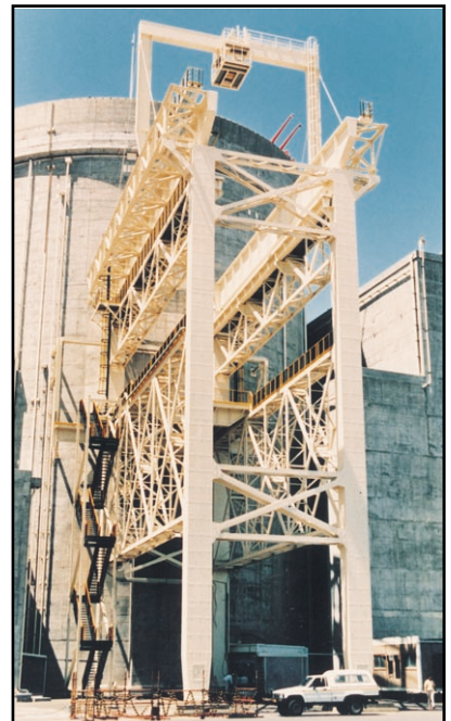
The completed Denso Steelcoat protection - maintenance free for 25-30 years.
