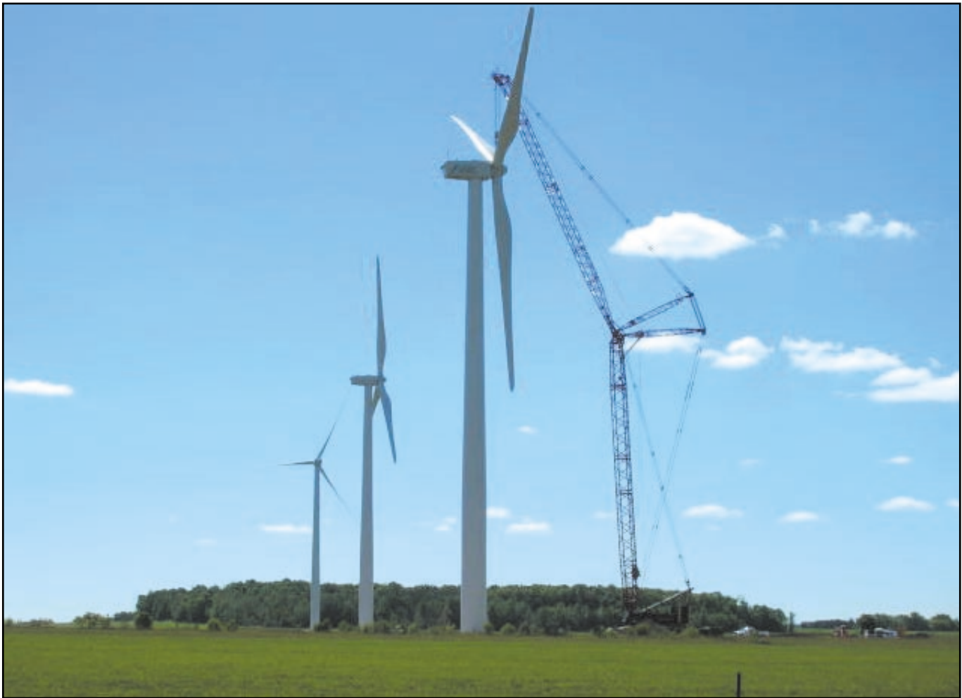
The Denso protected turbines under construction.
