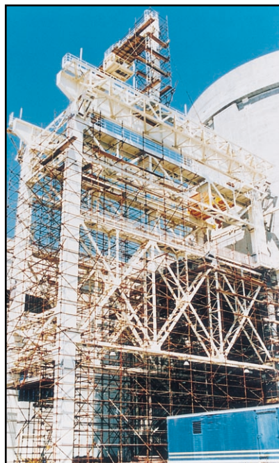
Denso Tape coating and overpainting with Denso Acrylic Topcoat in progress.
