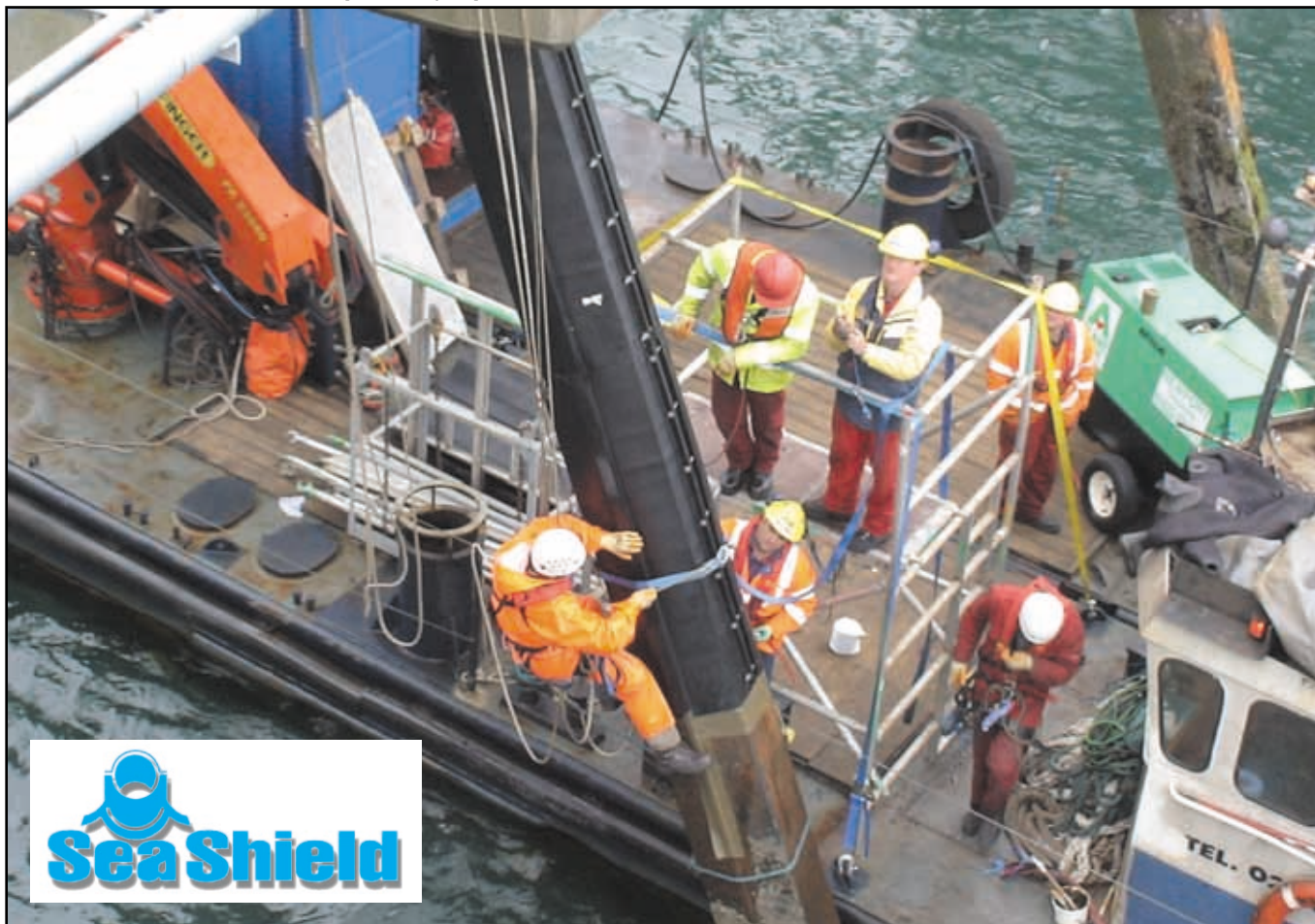
Below: Installation of SeaShield 2000HD on one pile is nearing completion.
