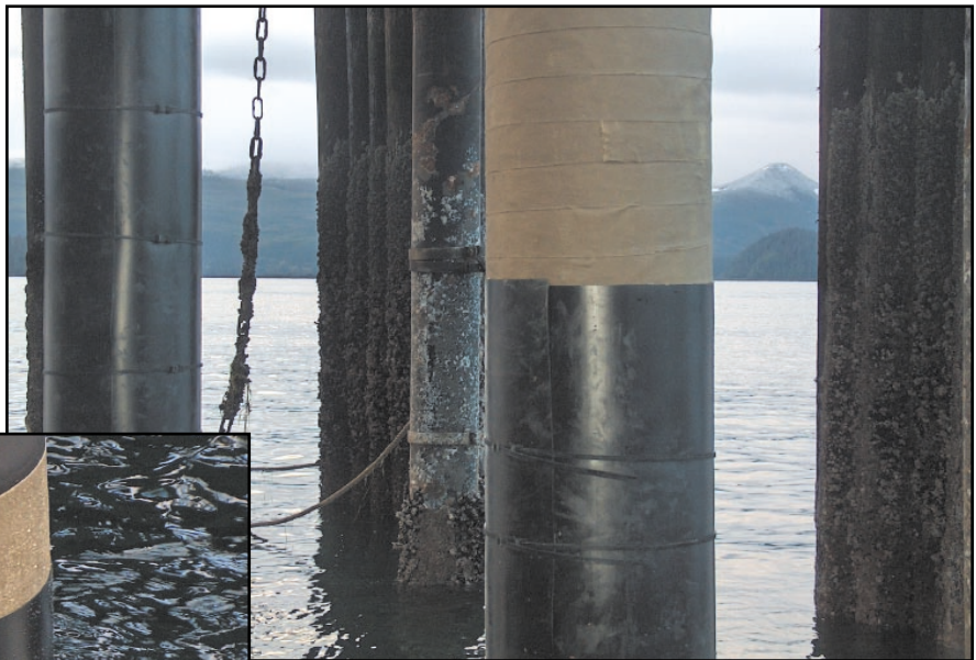
Above: center of picture shows Denso Marine Piling Tape protected pile with lower jacket in position.
