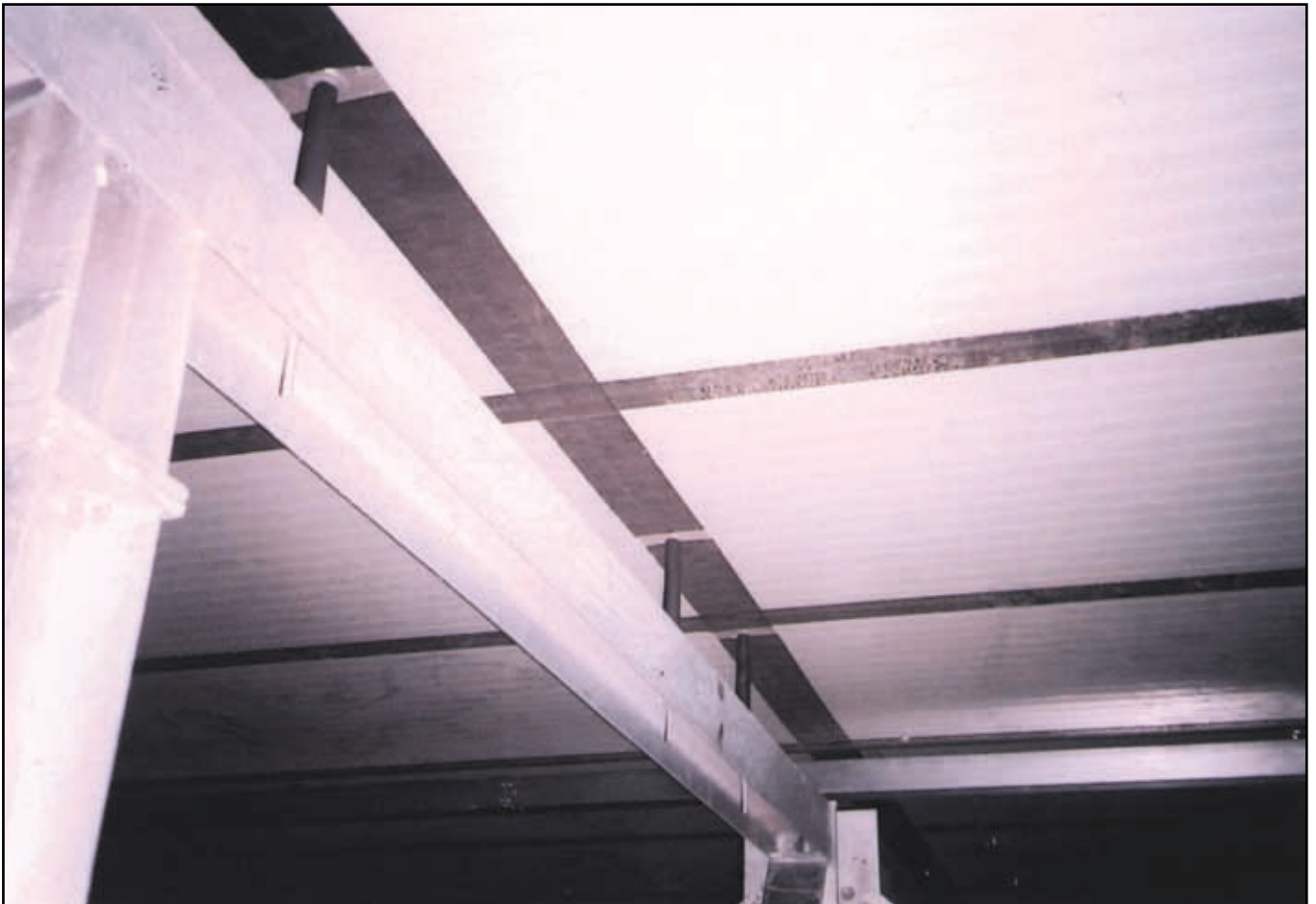
Coldstore insulation panels sealed with Denso Vapourseal Tape.
