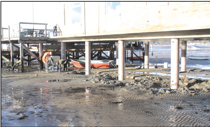
Installation of The SeaShield 500 system.
