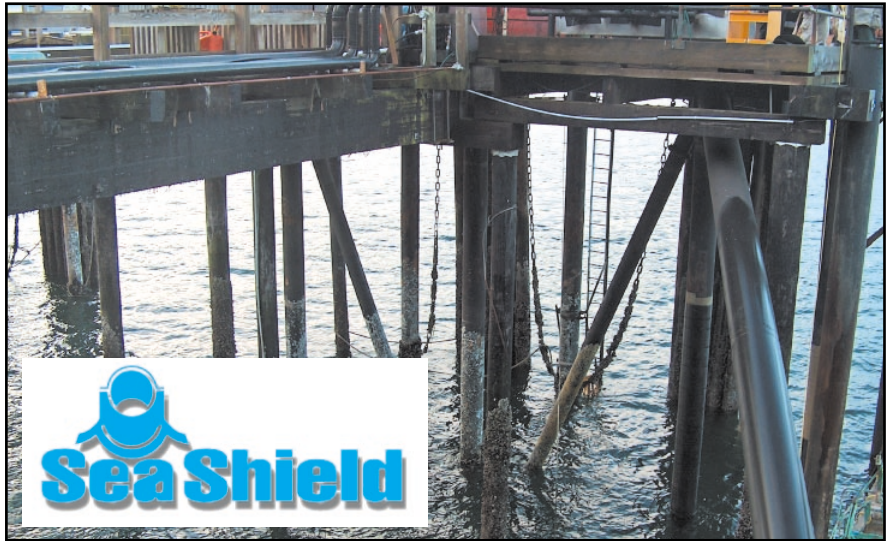
Above: The wharf is supported by 20 year old steel pilings.
