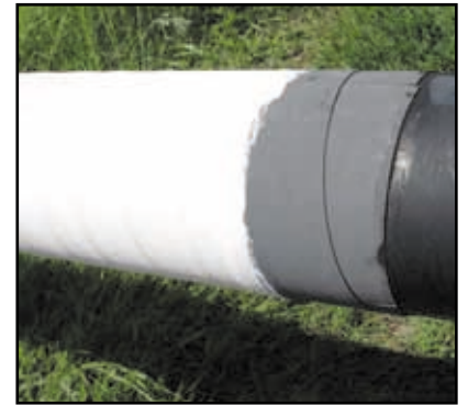
Above: To complete the System, a coat of the correct Denso Topcoat is applied over the Ultraseal Tape.
