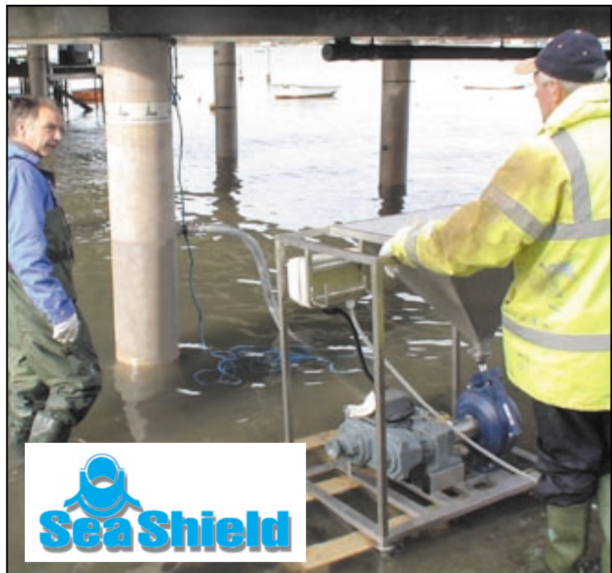
Below: The grout pump fills the fibreglass reinforced jacket with SeaShield 550 Epoxy Grout.
