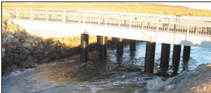
The Popes Nose Bridge with its SeaShield 100 Series protected piles.
