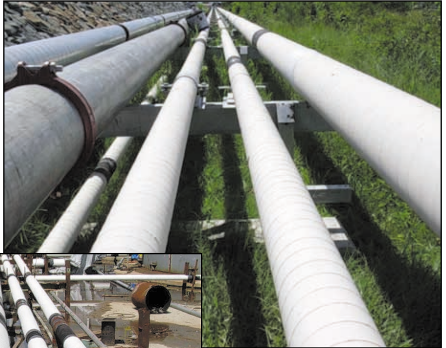
Above: To complete the System, a coat of the correct Denso Topcoat is applied over the Ultraseal Tape.
