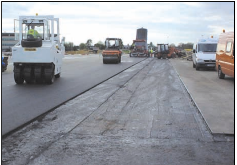
Above and below: The tarmacadam asphalt being laid up to the concrete slab on the right with Densoband used as a joint between the two areas.
