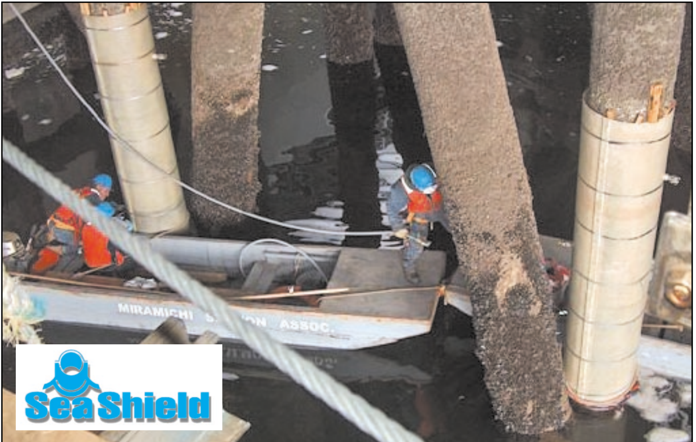
Installation of the SeaShield Series 500 system to eroded concrete marine piles on a jetty in the Bay of Fundy.
