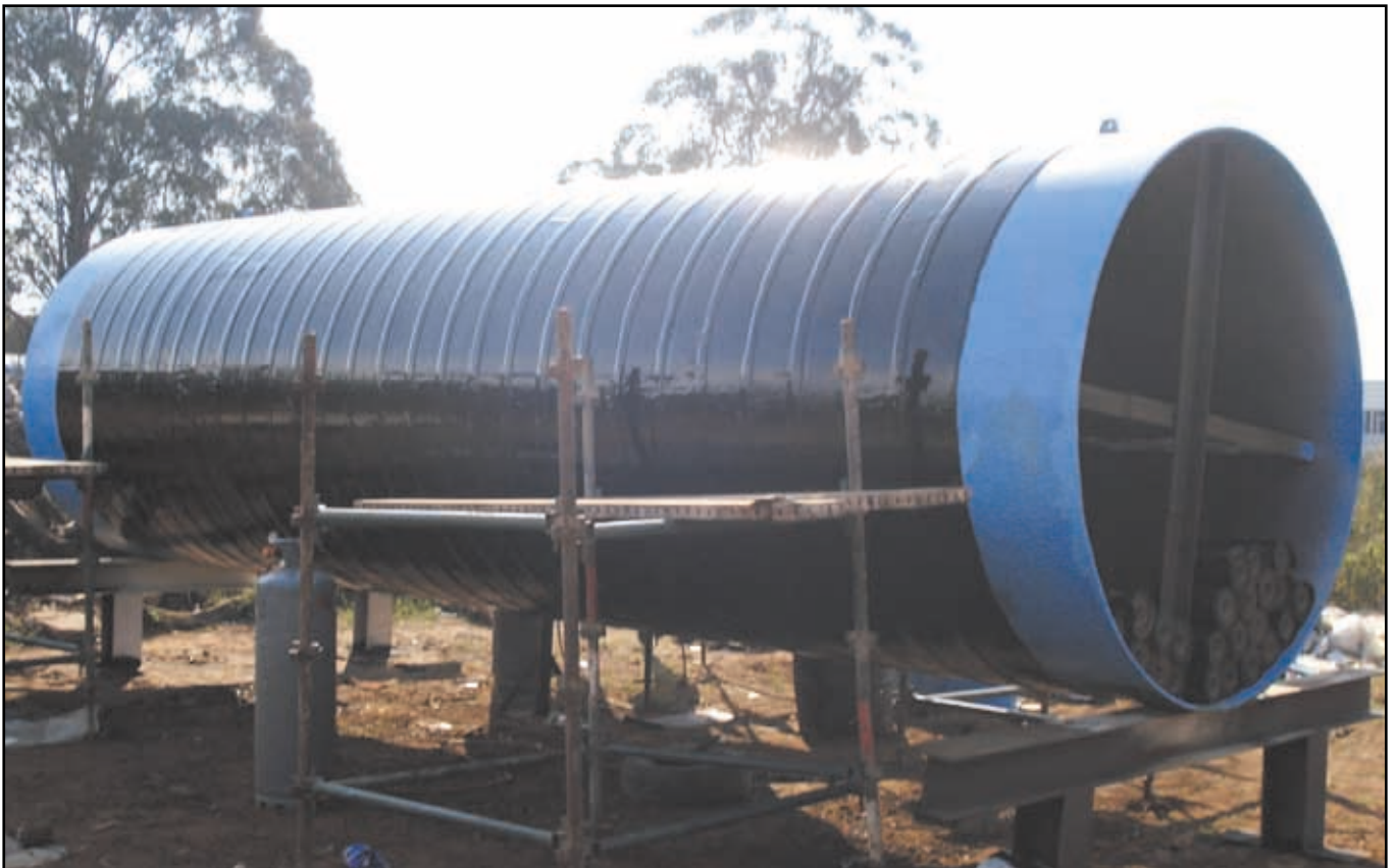
Above and below: Pipe sections were double wrapped with Densotherm HD at Gauteng before being transported to site.
