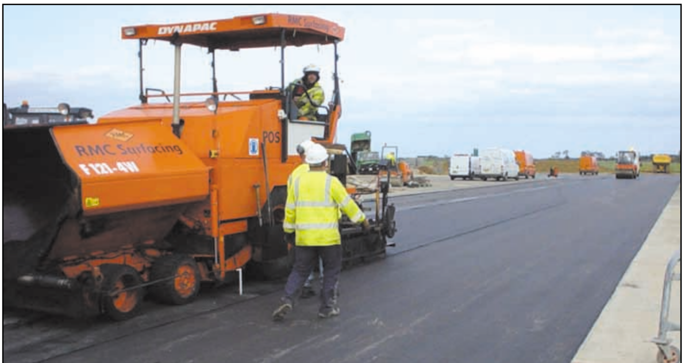
Above and below: The tarmacadam asphalt being laid up to the concrete slab on the right with Densoband used as a joint between the two areas.
