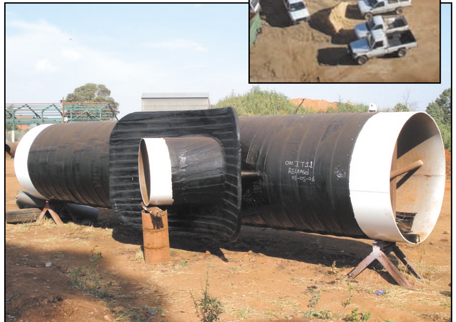
Above and below: Pipe sections were double wrapped with Densotherm HD at Gauteng before being transported to site.
