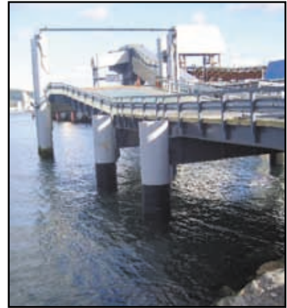
The Kaitaki Linkspan Berth in Wellington Harbour.
