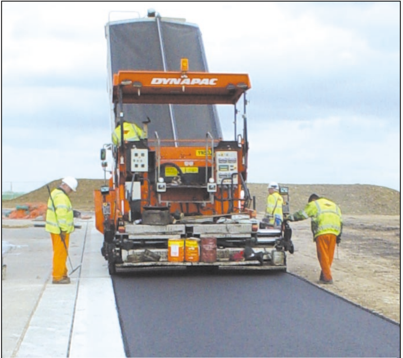
Densoband is used as a flexible joint between asphalt and concrete at East Midlands Airport - see page 3.
