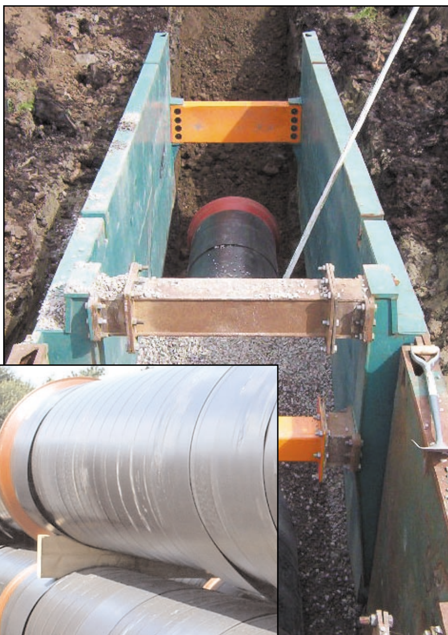
Above: Laying of the ductile iron pipeline in progress
