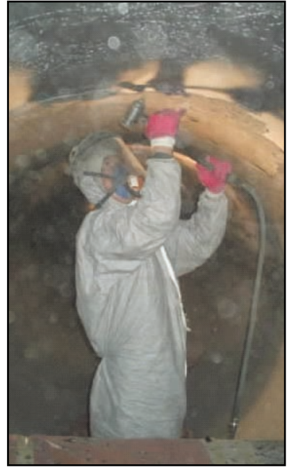
The old damaged epoxy lining being removed from the sea water pipe.
