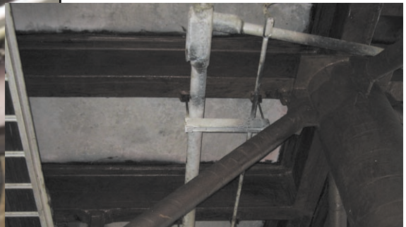
Above and left: Densyl Tape and Denso Hi-Tack Tape after 8 years service life.
