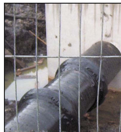
The completed P2 Densoclad protection.
