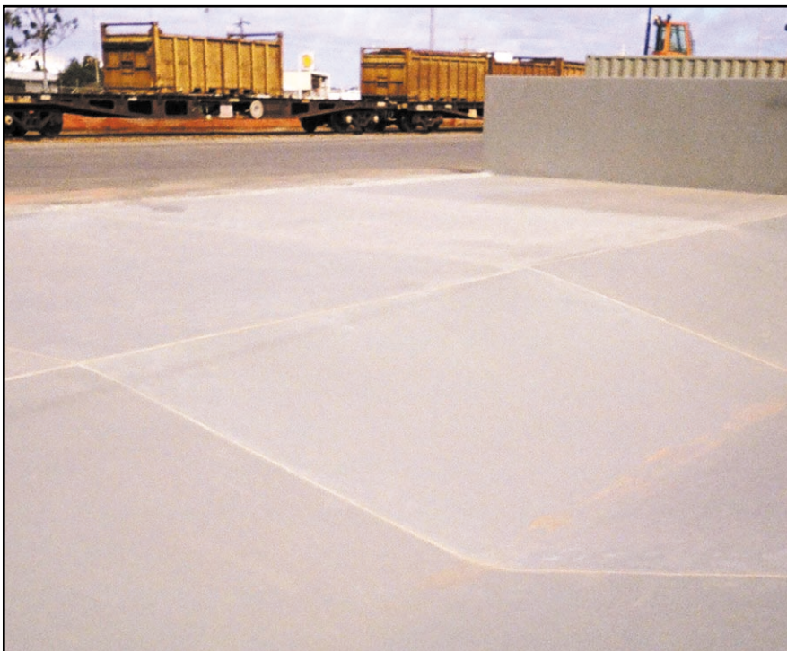
Above & below: The completed 'Dangerous Goods' bund area.
