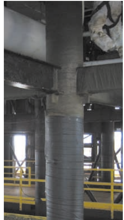
Above: Phase 2 - installation of Densyl Tape, Denso Hi-Tack Tape and Denso Utility Tape.
