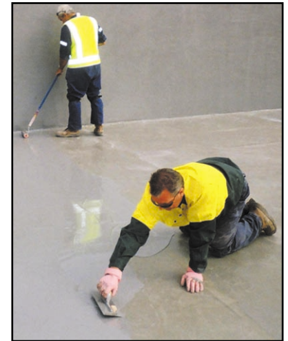
Above: Archco-Rigidon 703D system being applied to the concrete bund area.
