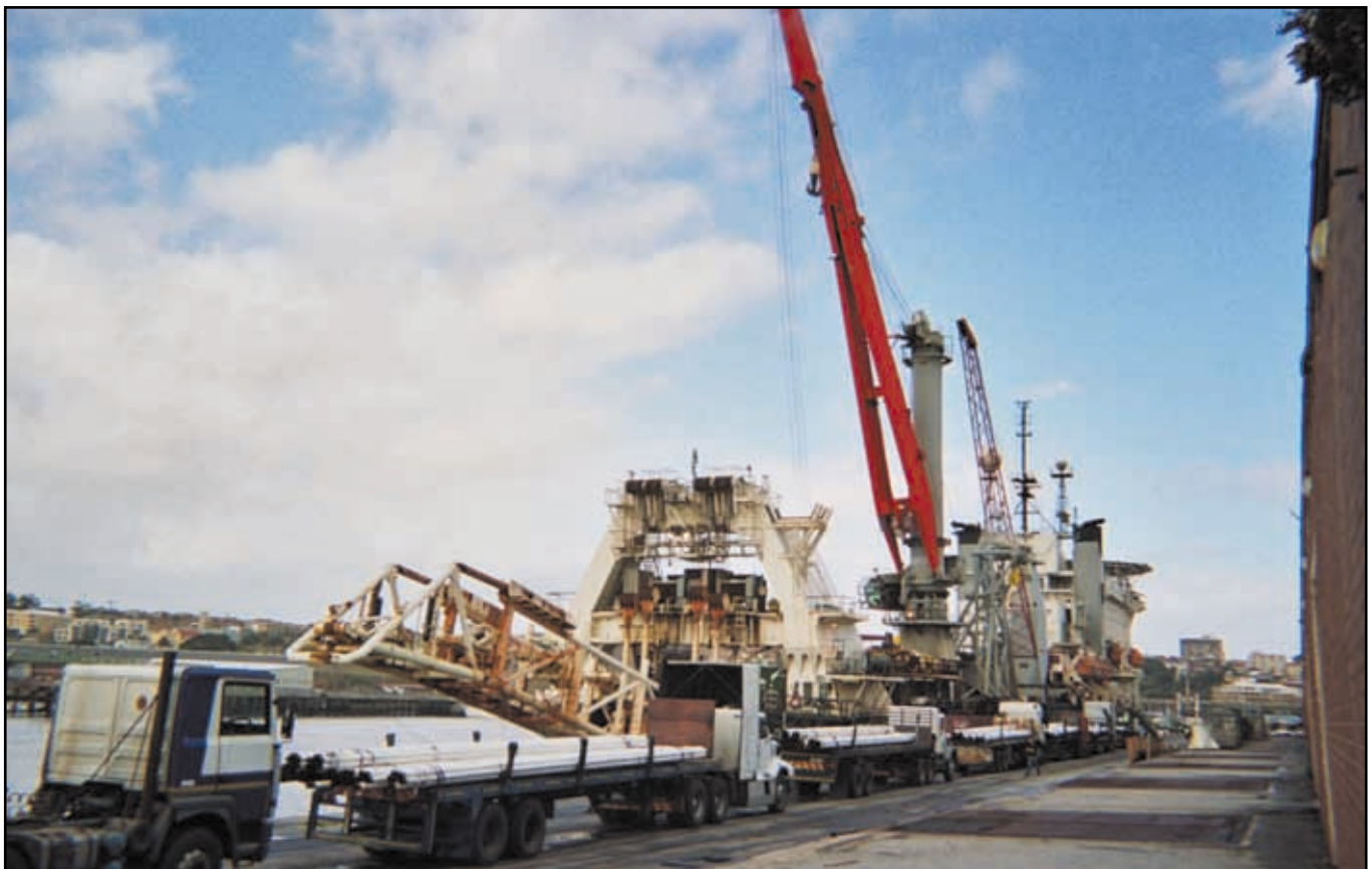
Below: The pipes being loaded onto the laybarge.
