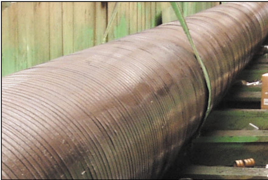
Above: 30" gas line protected with Protal 7250 overwrapped with Densopol Tape
