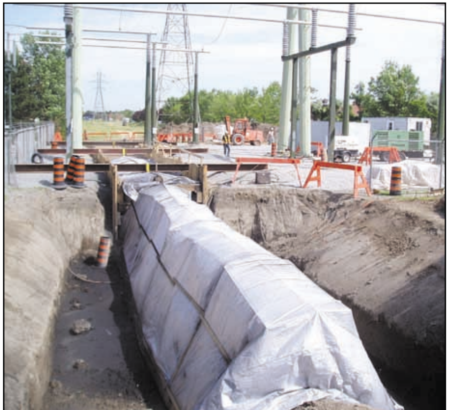
Above: 30" gas line protected with Protal 7250 overwrapped with Densopol Tape
