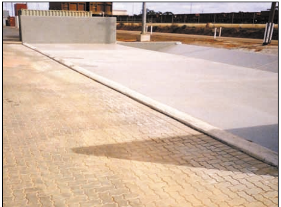
Above & below: The completed 'Dangerous Goods' bund area.
