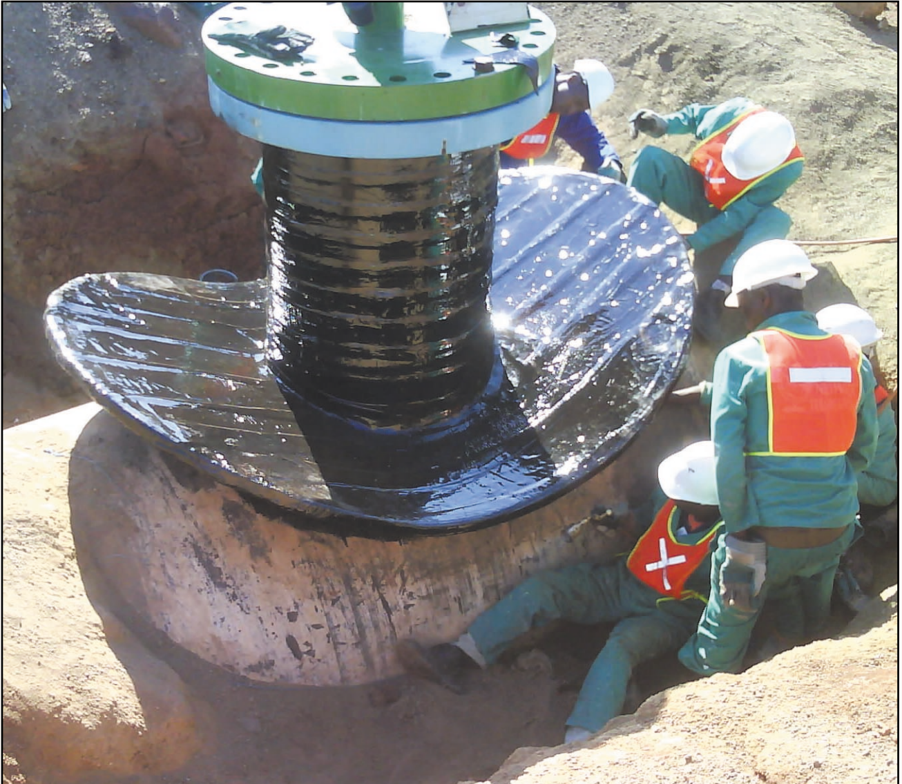
The Densotherm HD System used to protect a 1900mm x 800mm dia Crotch Plate Tee in South Africa - see page 11.
