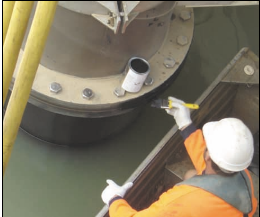
Above: Application of the Denso Butyl Primer to the cleaned flange crevice and edge.
