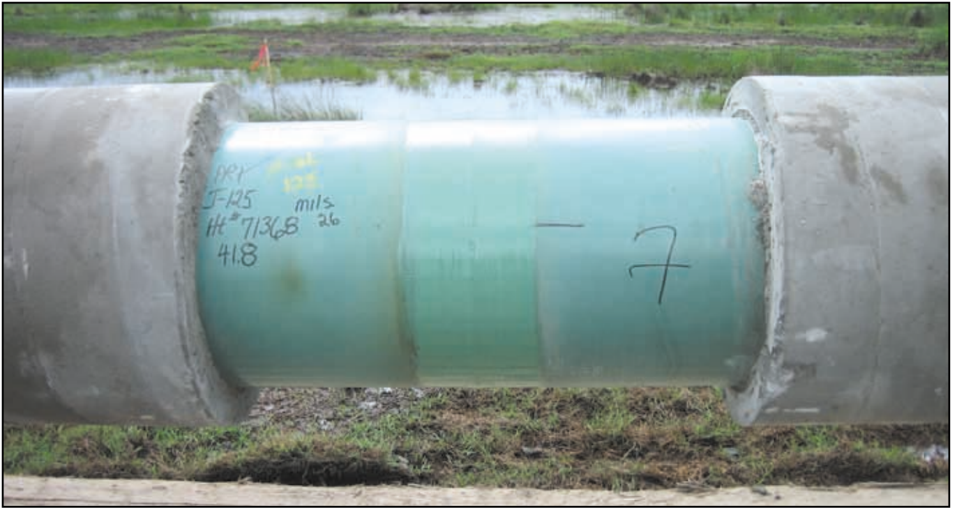
Above: Protal 7200 is cured and holiday detected within 15 minutes.
