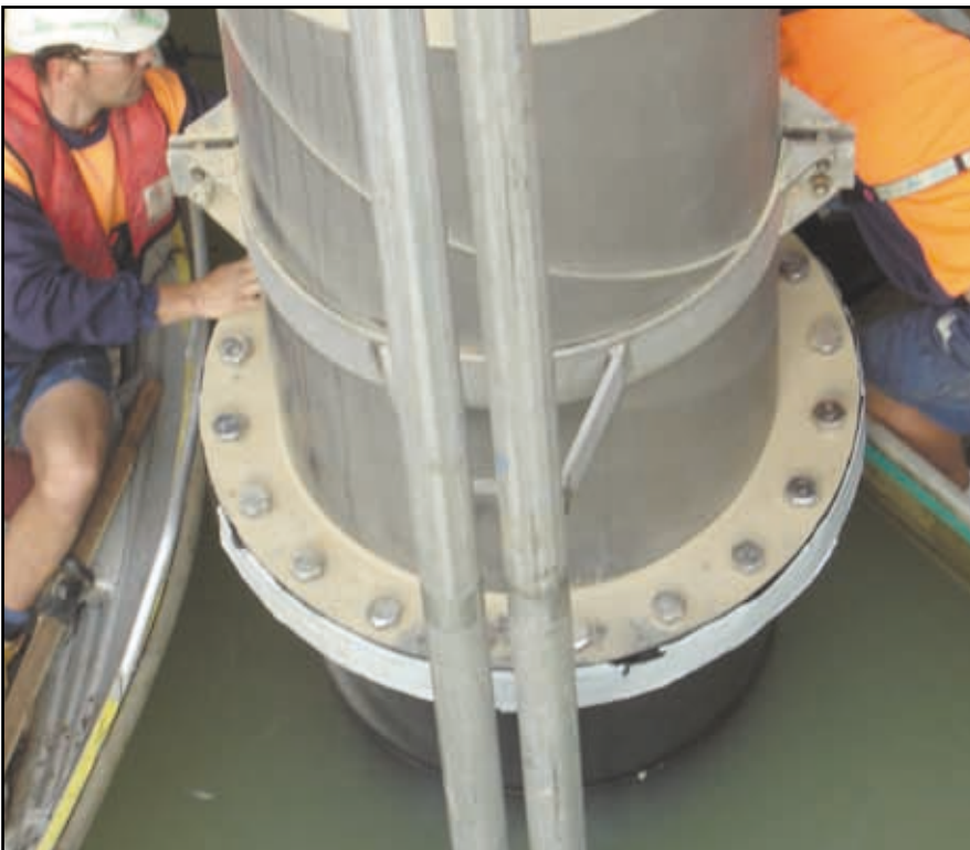
Above: Application of the Denso Butyl Primer to the cleaned flange crevice and edge.
