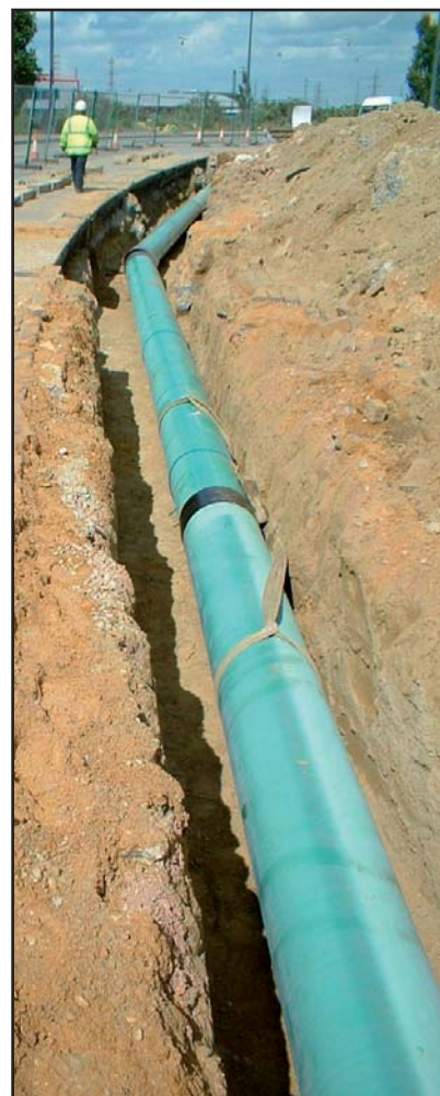
Morrison Utility Services PLC protected all joints and bends on the gas line with Densoclad 70 Tape. Denso Profiling Mastic was used to fill voids etc before wrapping.
