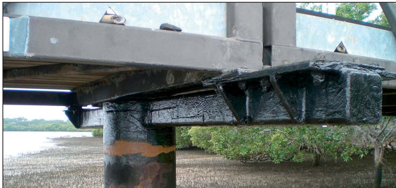
Above: Priming with Denso Hi-Tack Primer after cleaning with hand power tools.
