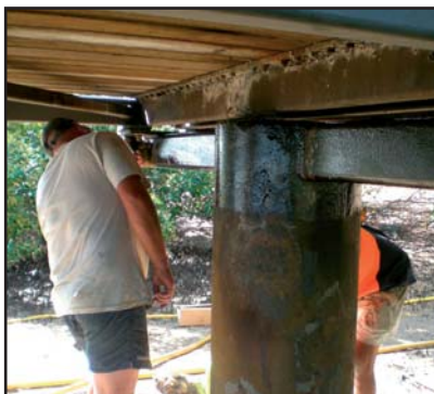
Above: Priming with Denso Hi-Tack Primer after cleaning with hand power tools.
