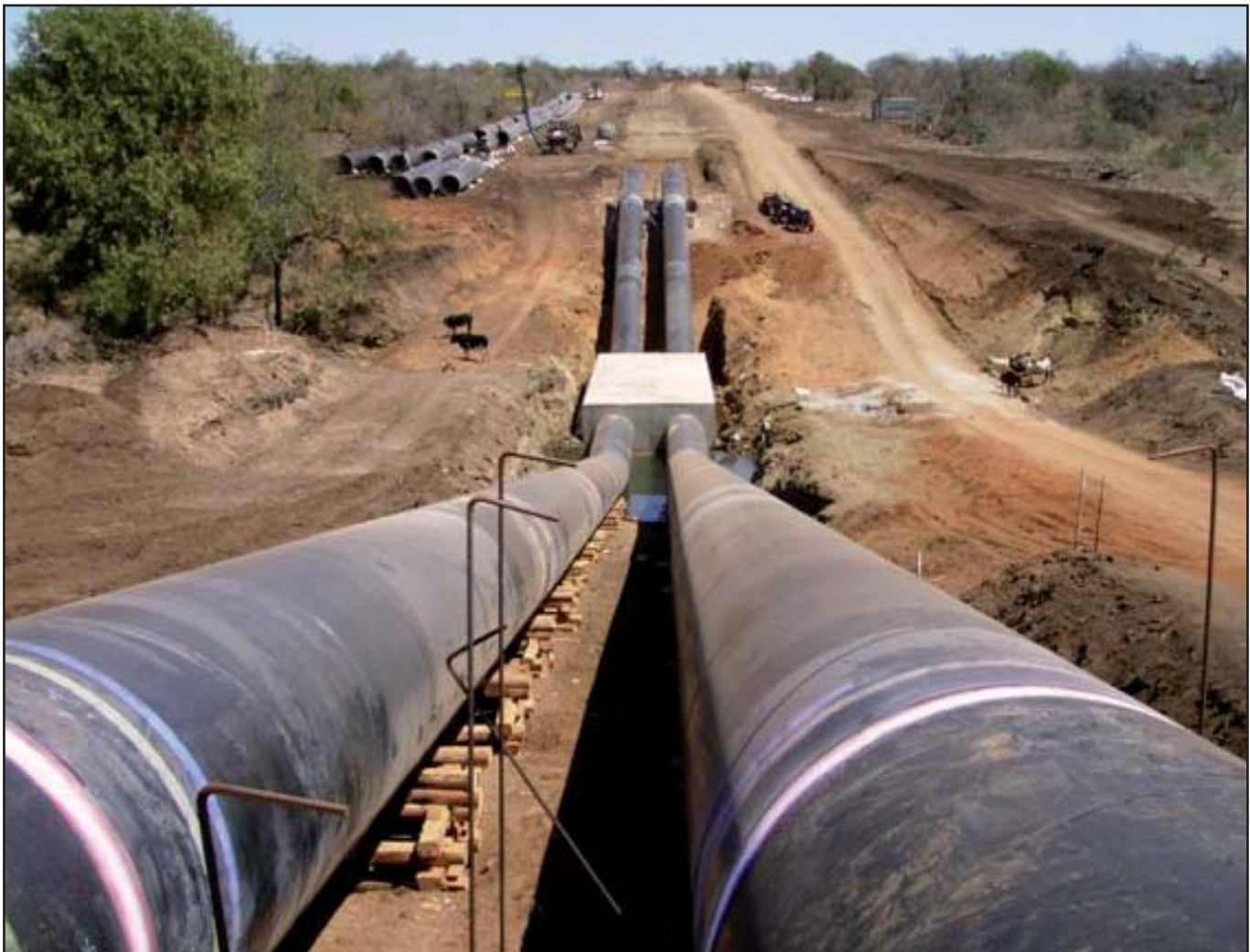
Below: View of the LUSIP project during construction.
