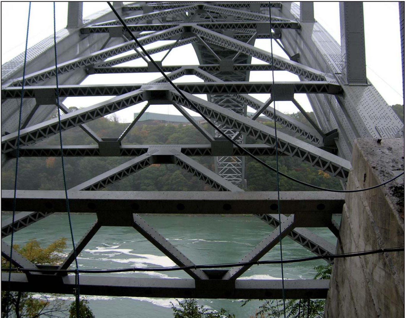
Below and opposite: Various views of the Rainbow Bridge that crosses from Canada to the USA.
