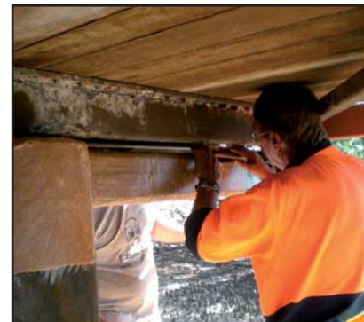
Above: Taping with Denso Hi-Tack Tape
