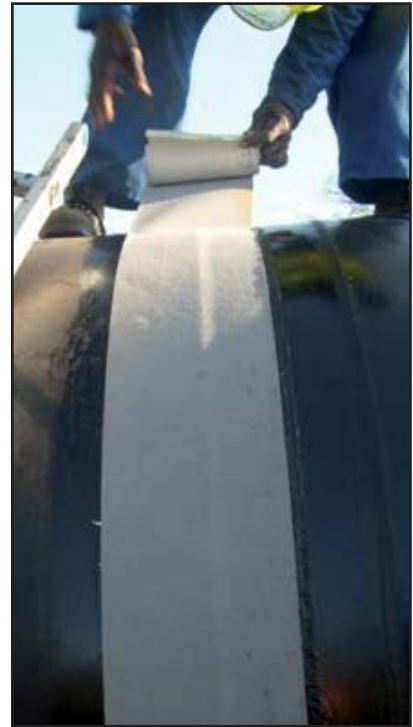
Above: Application of the Denso Steelcoat 500 System to the exposed irrigation pipeline field joints.
