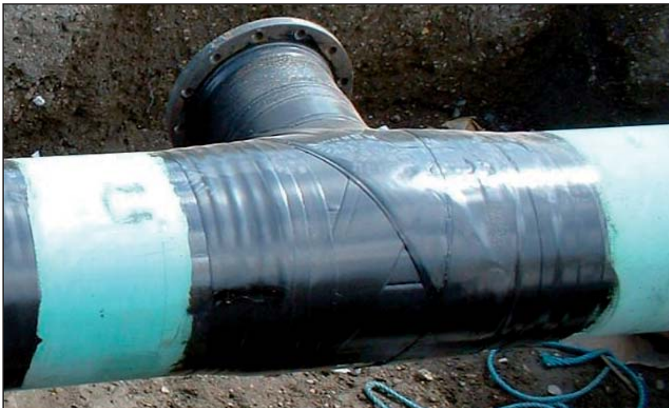
Morrison Utility Services PLC protected all joints and bends on the gas line with Densoclad 70 Tape. Denso Profiling Mastic was used to fill voids etc before wrapping.
