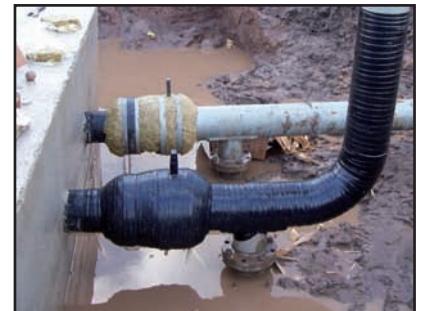
Above: The application of Denso Profiling Mastic. Below: Flange overwrapped with Densoclad 70 Tape.
