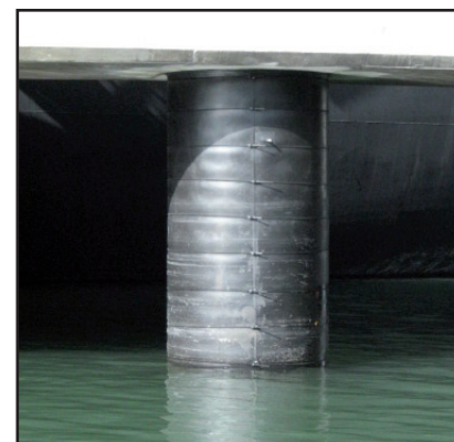
Pictures: Seashield Series 100 system protects more than 100 tubular steel piles at the Kooragang Terminal.
