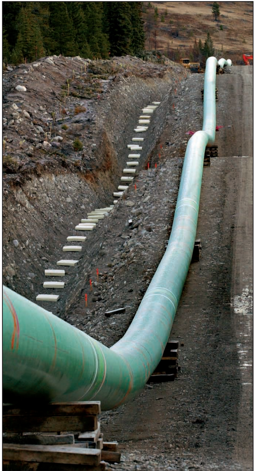
The pipelengths are welded together and the welded joint areas are then coated with Denso Protal 7200 before being buried.
