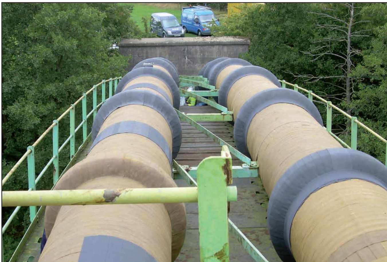
After the Denso Hi-Tack Tape is applied to the 33" water main, the joints are overwrapped with Denso Ultraseal Tape.
