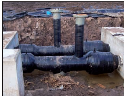
The protected flange joints prior to burial.
