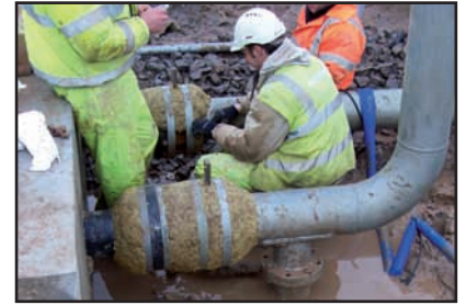
Above: The application of Denso Profiling Mastic. Below: Flange overwrapped with Densoclad 70 Tape.
