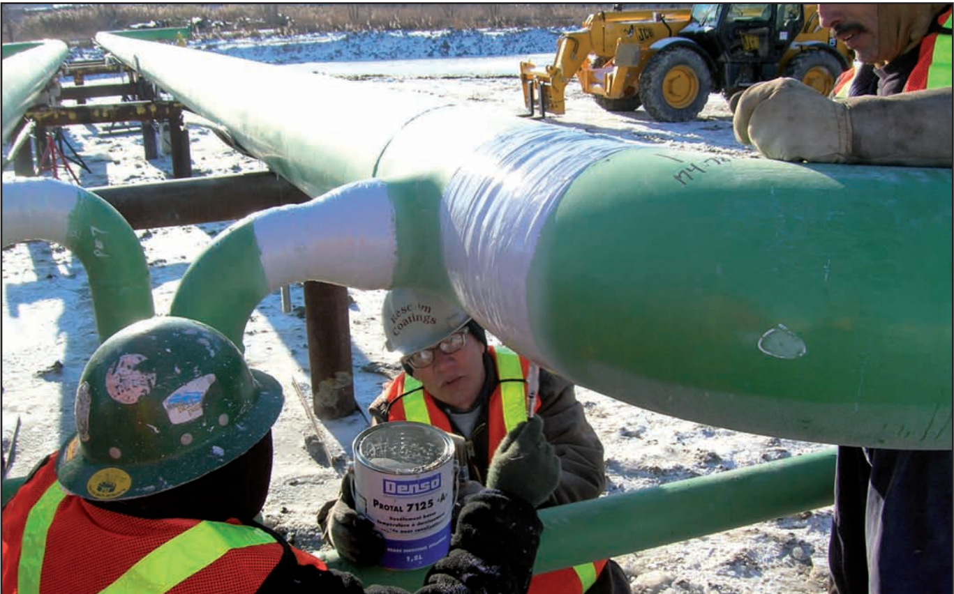
Above and below: With no preheating necessary, the girth welds can easily be coated with Protal 7125 at temperatures of -15^{\circ}\text{C} . Inset above: New jet fuel tanks being constructed approximately 5km from the airport
