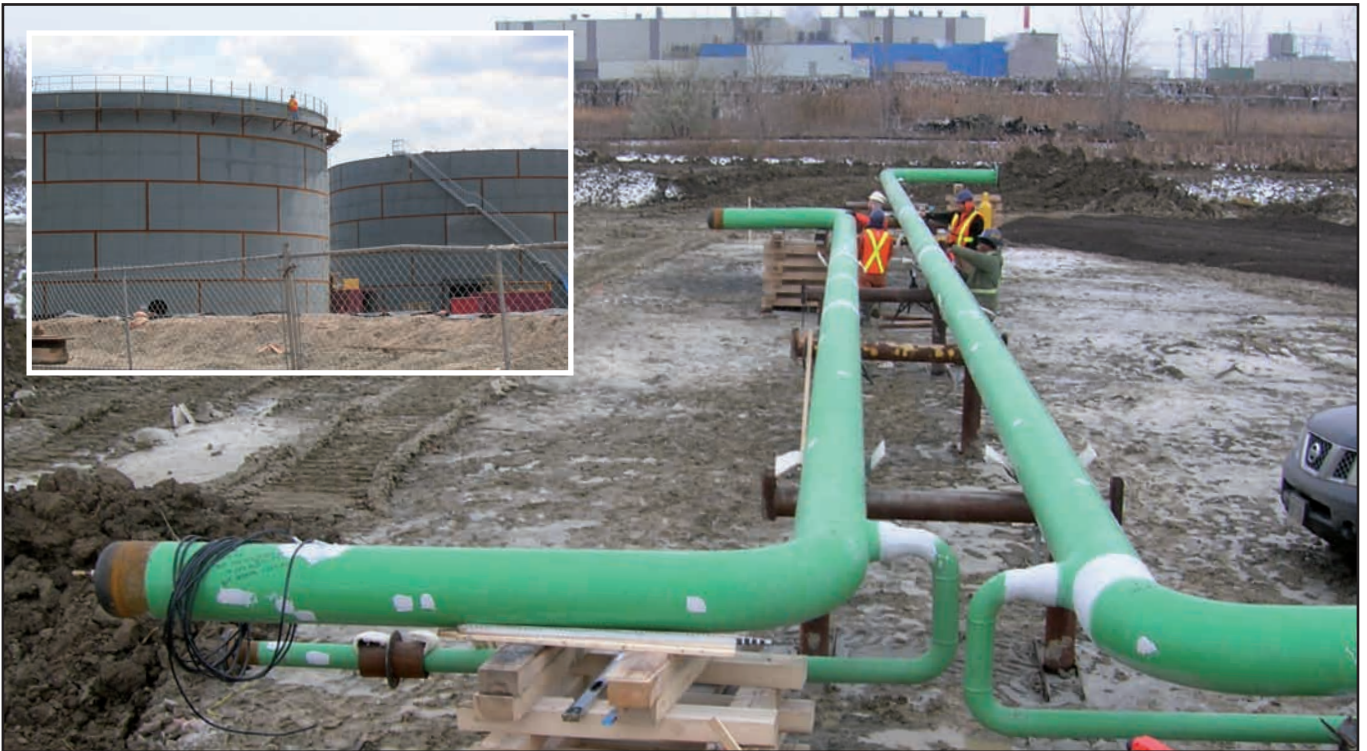
Above and below: With no preheating necessary, the girth welds can easily be coated with Protal 7125 at temperatures of -15^{\circ}\text{C} . Inset above: New jet fuel tanks being constructed approximately 5km from the airport
