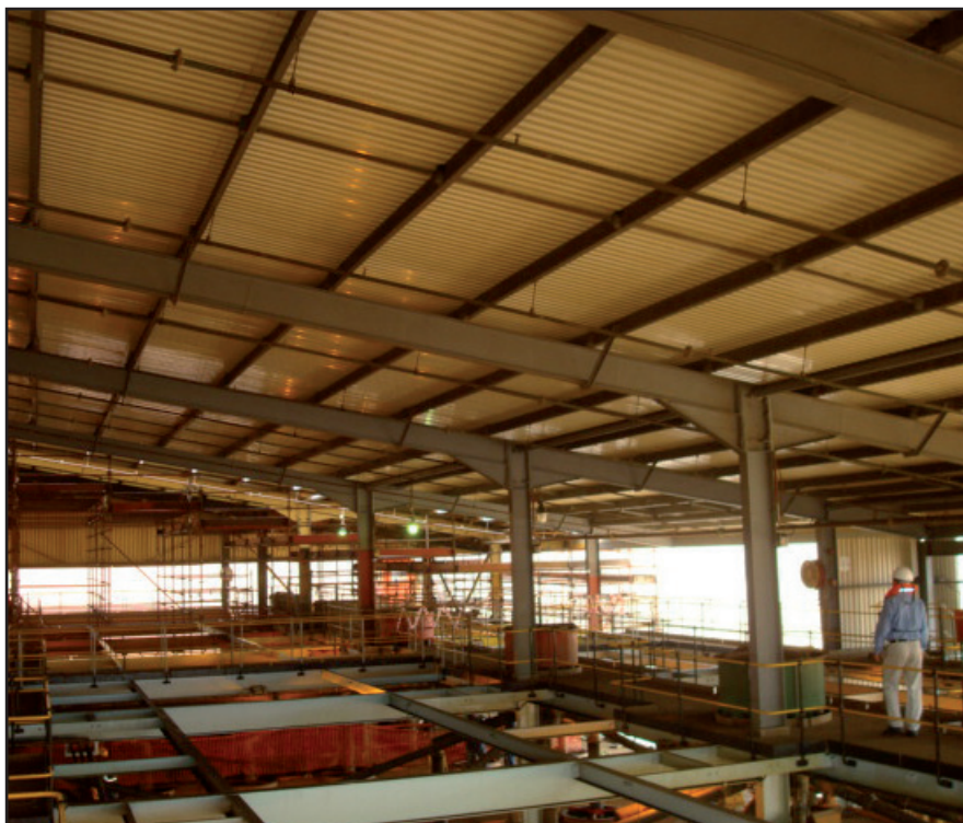
The roof structure of the dredger is protected against the highly corrosive environment with the Denso Steelcoat 400 System.
