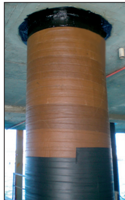
Above: Application of the SeaShield 80 System underway showing completed Steelcoat 100 System at the top of the pile.
