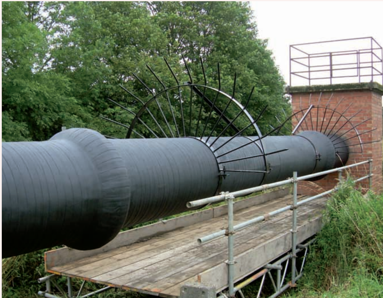
Denso Steelcoat 400 and 700 Systems used on the Ercebridge pipebridge near Darlington - see story pages 4-5.
