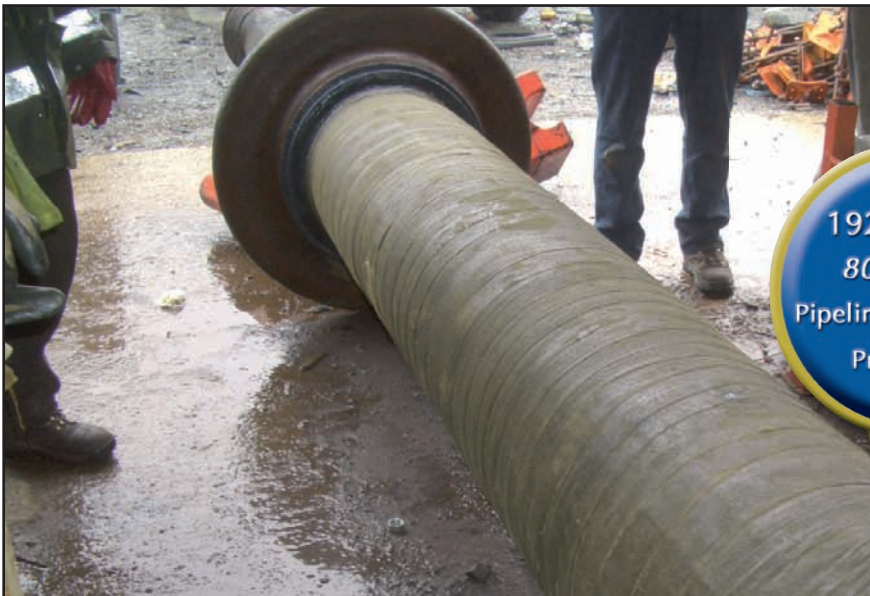
The original crane pillar is coated with Denso Paste before being wrapped with Denso Tape.
