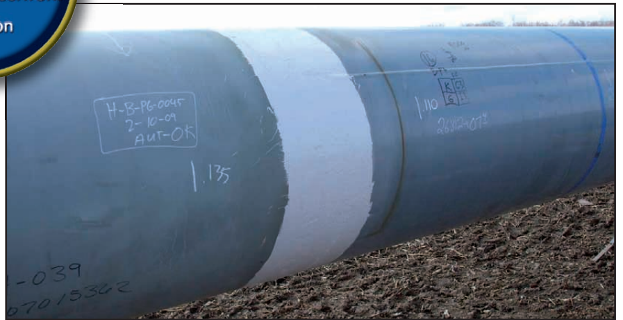
Above: Applying Protal 7125 at 50 mils for directional drill on 42" diameter pipe. Below: Coated girth weld with Protal 7125
