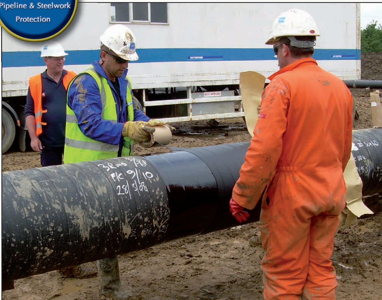
Densoclad Tape protecting pipes in a corrosive brine field environment - see story page 4.
