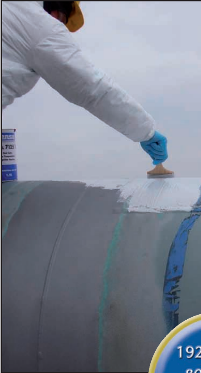
Applying Protal 7125 by brush.
