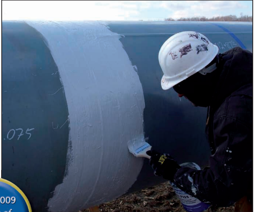
Above: Applying Protal 7125 at 50 mils for directional drill on 42" diameter pipe. Below: Coated girth weld with Protal 7125
