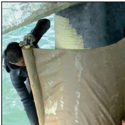
4. A single sheet of Denso Hi-Tack Tape is then positioned as a band, over the Densyl Tape and around the whole pile.
