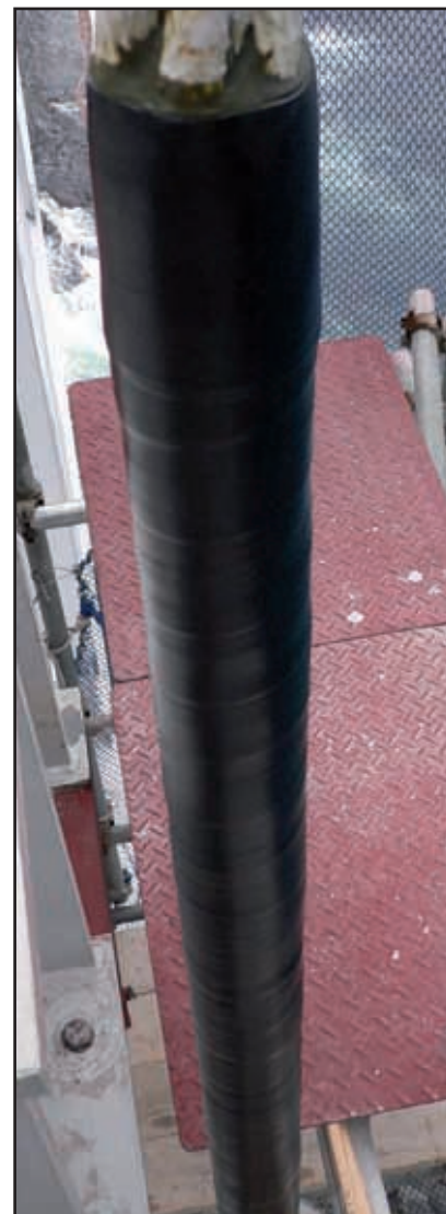
3. A final wrap of self-adhesive tape completes the protection system.
