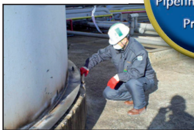
2. Preparation - cleaning the area ready for the Denso system.
