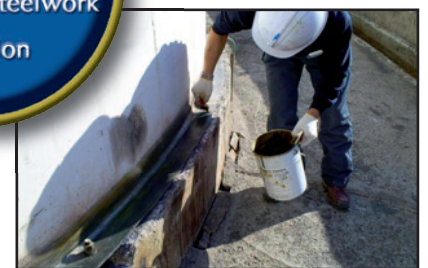
3. Priming the steel surfaces with Denso Hi-Tack Primer.
