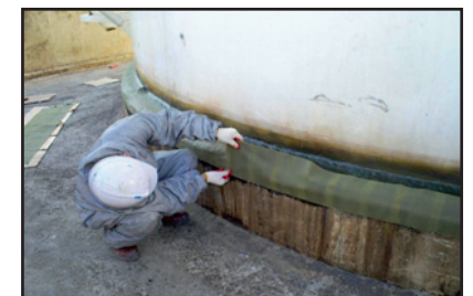
6. Applying the Densyl KF Tape to complete the system.
