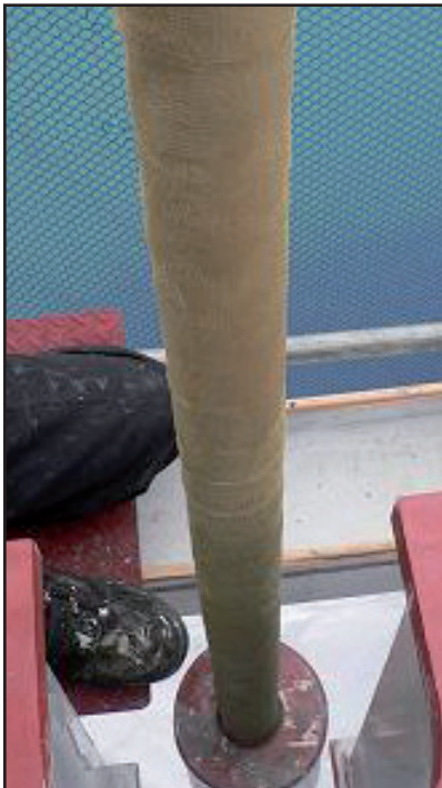
2. After applying a coating of Denso Paste, over the Densyl Mastic Strips and cable strands, Densyl KF Tape is spirally wrapped with a 55% overlap.
