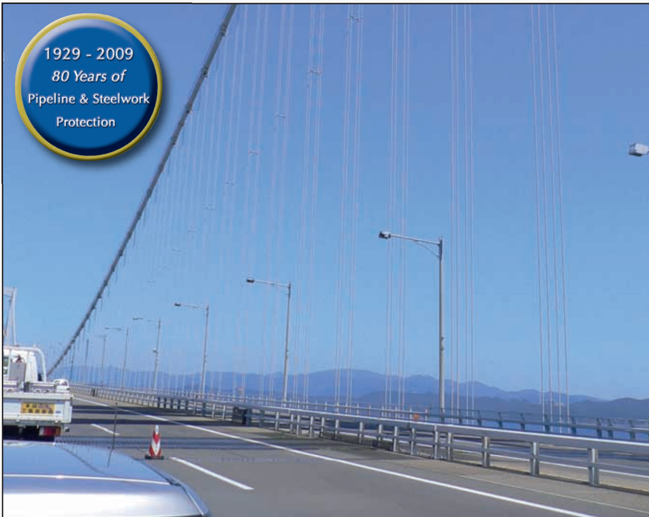
A Denso System protects the suspension cables on the Ohmishima Great Bridge, Japan - see story page 11.
