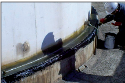
4. Priming the concrete surfaces with Denso Primer D.
