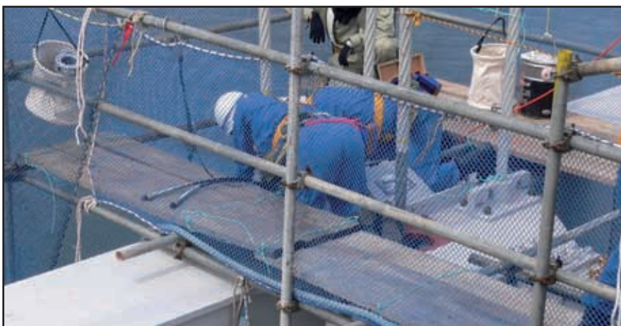
Cable protection work in progress on the Ohmishima Great Bridge.
