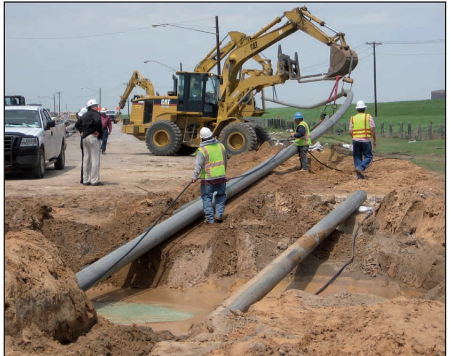
Photos: Above: Directional drill application with Protal ARO coated pipe. Below: Protal ARO being spray applied in the shop
