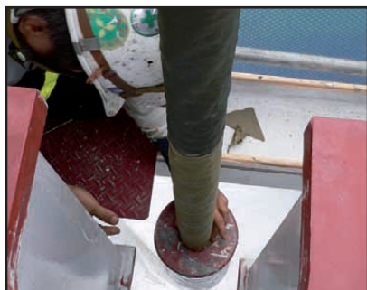
2. After applying a coating of Denso Paste, over the Densyl Mastic Strips and cable strands, Densyl KF Tape is spirally wrapped with a 55% overlap.
