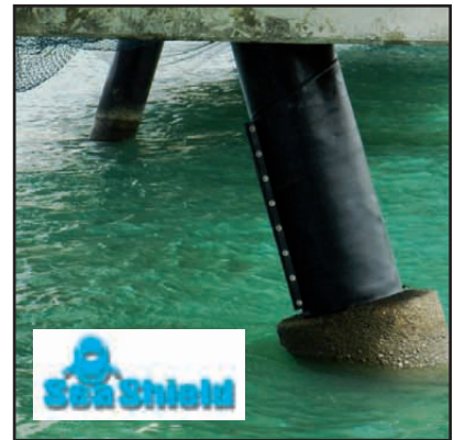
6. The finished application, a durable and neat repair for the damaged piles.
