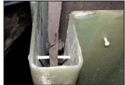
3. Annulus space adjusted with plastic screws between Fiber-Form and H-pile.
