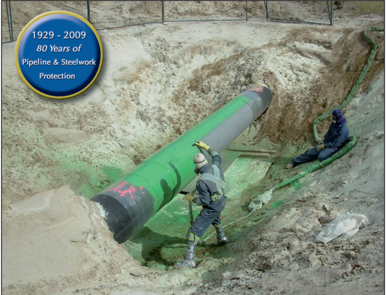
Denso Protal 7250 being applied to a crude oil pipeline in Canada - see story page 6-7.
