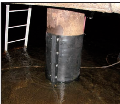
Completed installation of SeaShield 2000FD on 18" diameter pile.
