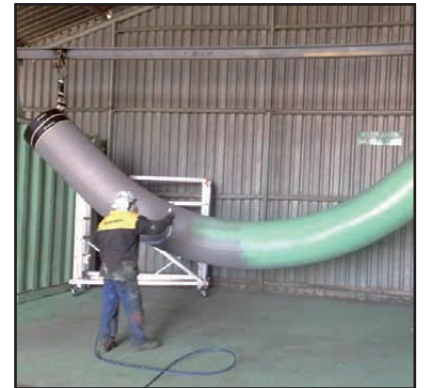
A pipeline bend being spray coated with Denso Protal 7200.
