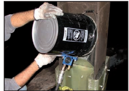
4. Pouring of mixed Seshield 550 Epoxy Grout through pneumatic vibratory funnel.
