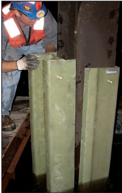
1. Installation of the two Fiber-Form half shells.
