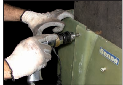
2. Installation of the screws through the tongue and groove closure.
