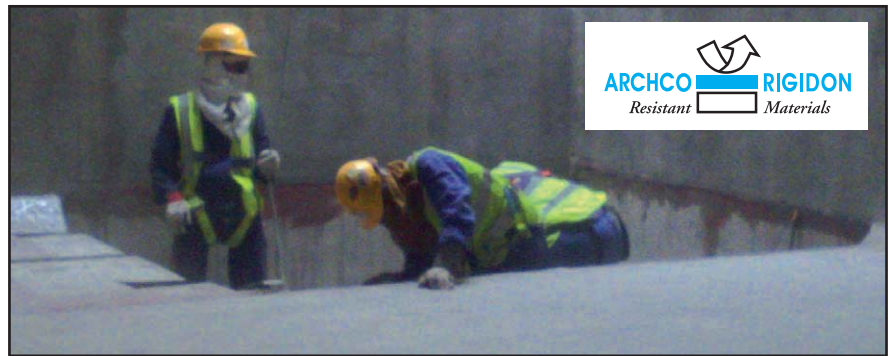
Above and Below: Archco-Rigidon 623D and 603D linings were applied to the floors and walls of the concrete neutralisation tanks. The Archco-Rigidon 603D lining was used on the manhole covers.
