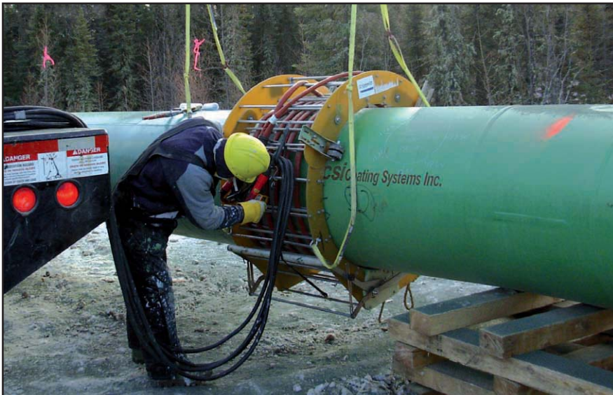
Setting up a heat induction coil
