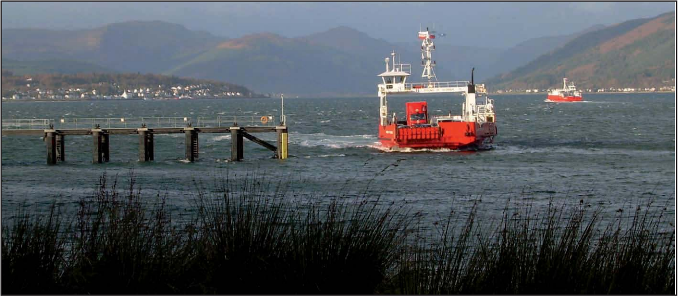
Above and Below: A car ferry approaching the new berthing structures located at McInroy's Point, Firth of Clyde.
