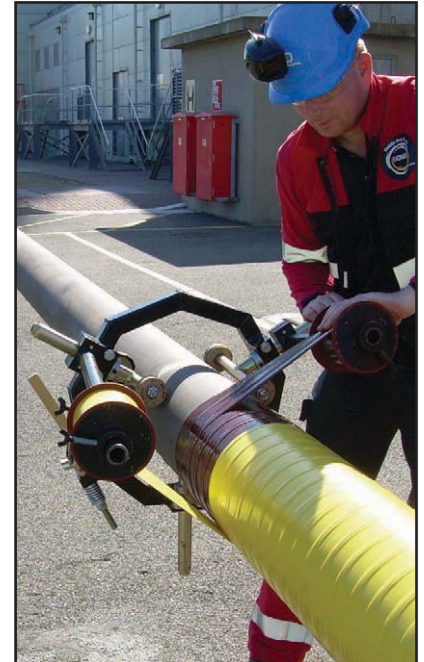
The perfect dual application of Denso Hotline Tape and Denso Self-adhesive PVC Tape is achieved in one easy operation using a Denso Hand Wrapping Machine.
