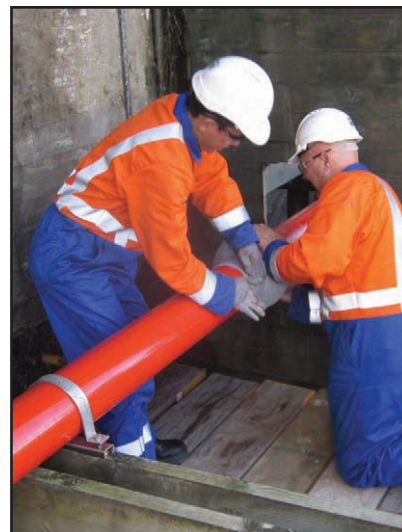
Application of the Denso KF Colourtape.
