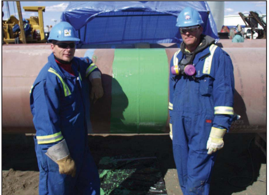
The highly skilled crew from Ledcor with a recently completed a Protal 7200 protected joint.
