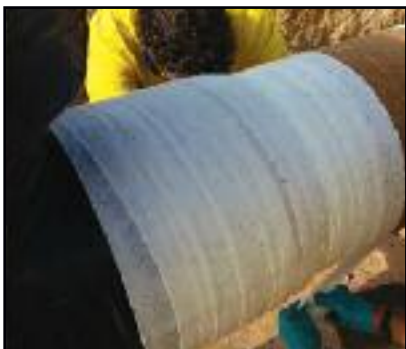
Application of the Glass Outerwrap System.
