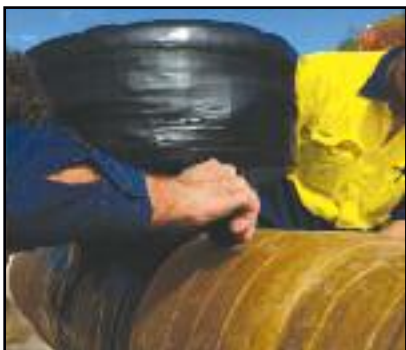
Application of the SA PVC Tape.
