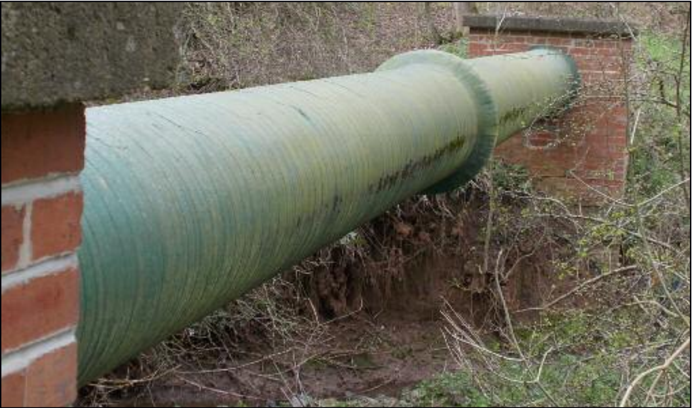
Above: The original 2005 applied Steelcoat 400/100 System. The photo was taken in 2016 showing a little moss and dirt accumulation as to be expected.
