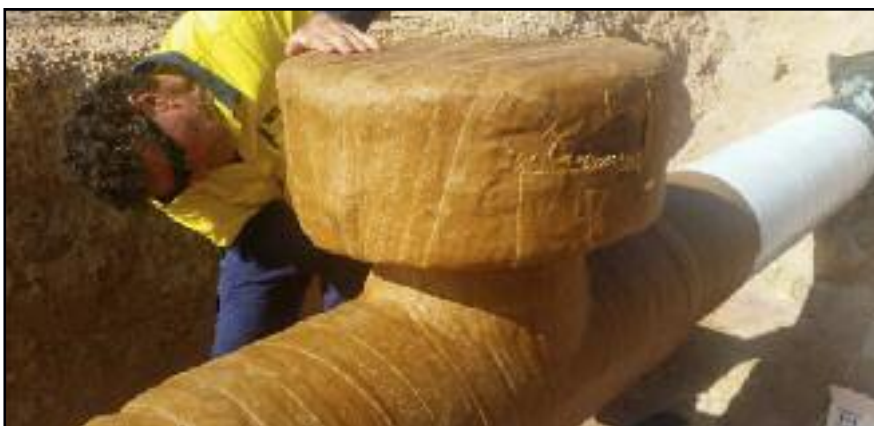
Application of the Denso Petrolatum Tape System.
