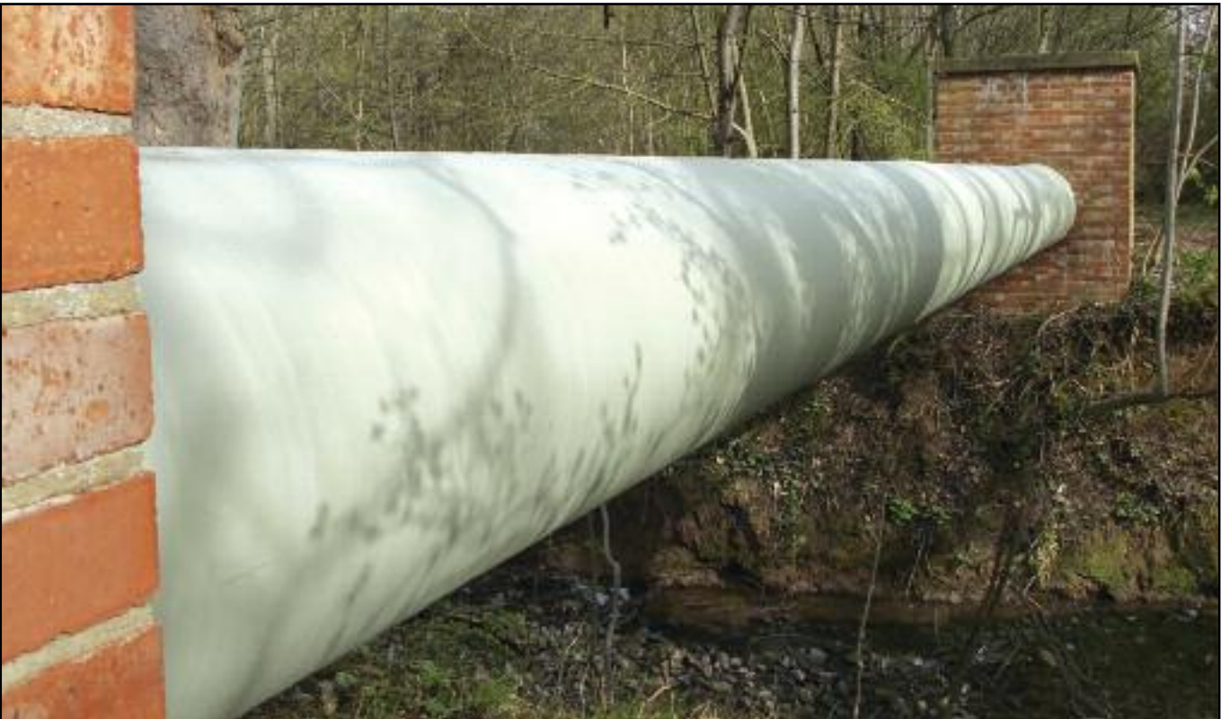
Below: The completed 2016 Steelcoat 400/100 System in sage green finish.
