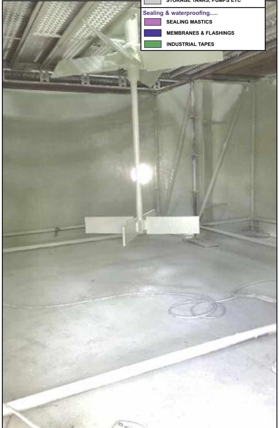
The Cristal mixer tank lined with Archco-Rigidon 403D by Hertel (UK).
