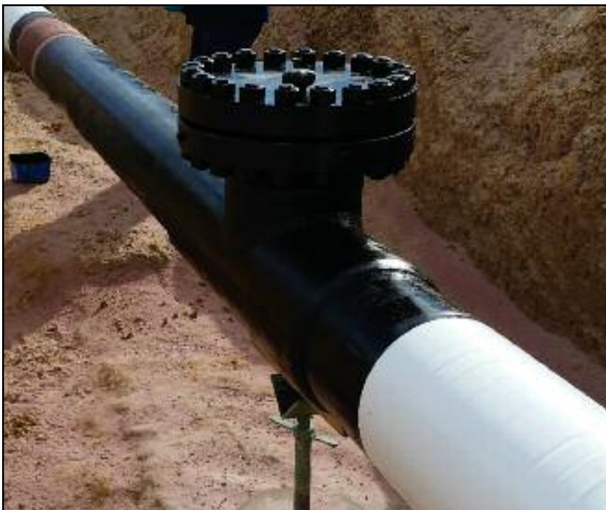
Protection of a joint and tie-in to existing coating underway.
