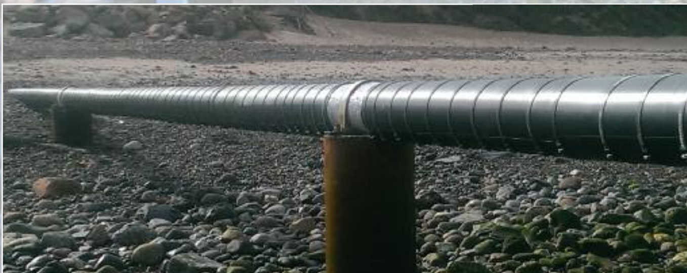
Above: Damage to the cement mortar on the Jurby outfall pipe.
