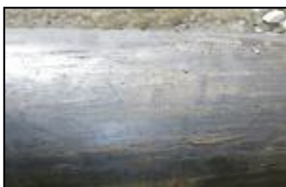
The pipe still in perfect condition - immediately after the removal of the original Denso system and still showing a layer of petrolatum compound.
