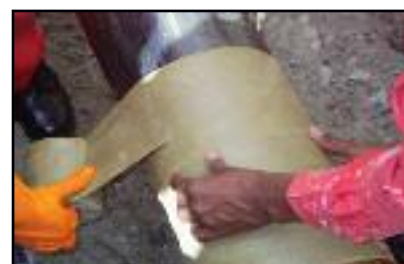
After cleaning, the pipe was re-coated with the Denso Petrolatum Tape System using a 55% overlap of the tape.
