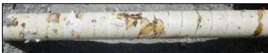
The original outer wrap damage was partly caused by the backfills and recent excavation.
