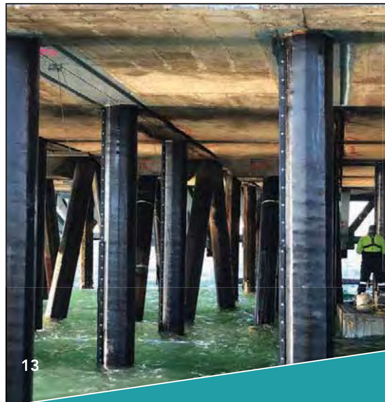
View underneath the BlueScope Wharf showing the installation of the SeaShield 2000FD™ system to the steel piles.
