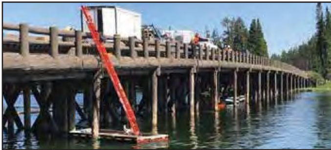
Contractor preparing deteriorated timber piles for the installation of Denso's SeaShield Series 500™ Fiber Glass Jacket System
