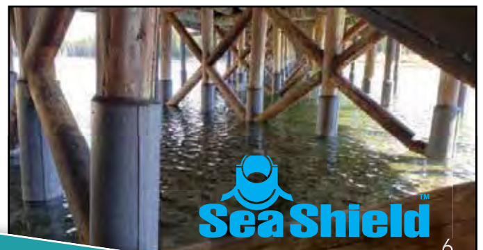
Timber piles fully protected using the SeaShield Series 500™ System from weathering and deterioration.
