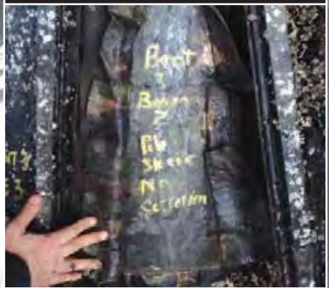
SeaShield protected pile inspected and showing no corrosion after 10 years service.
