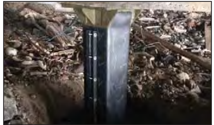
Below: Steel cross beams protected with Denso Glass Outerwrap 70™ in lieu of the 80 mil HDPE Outercovers.
