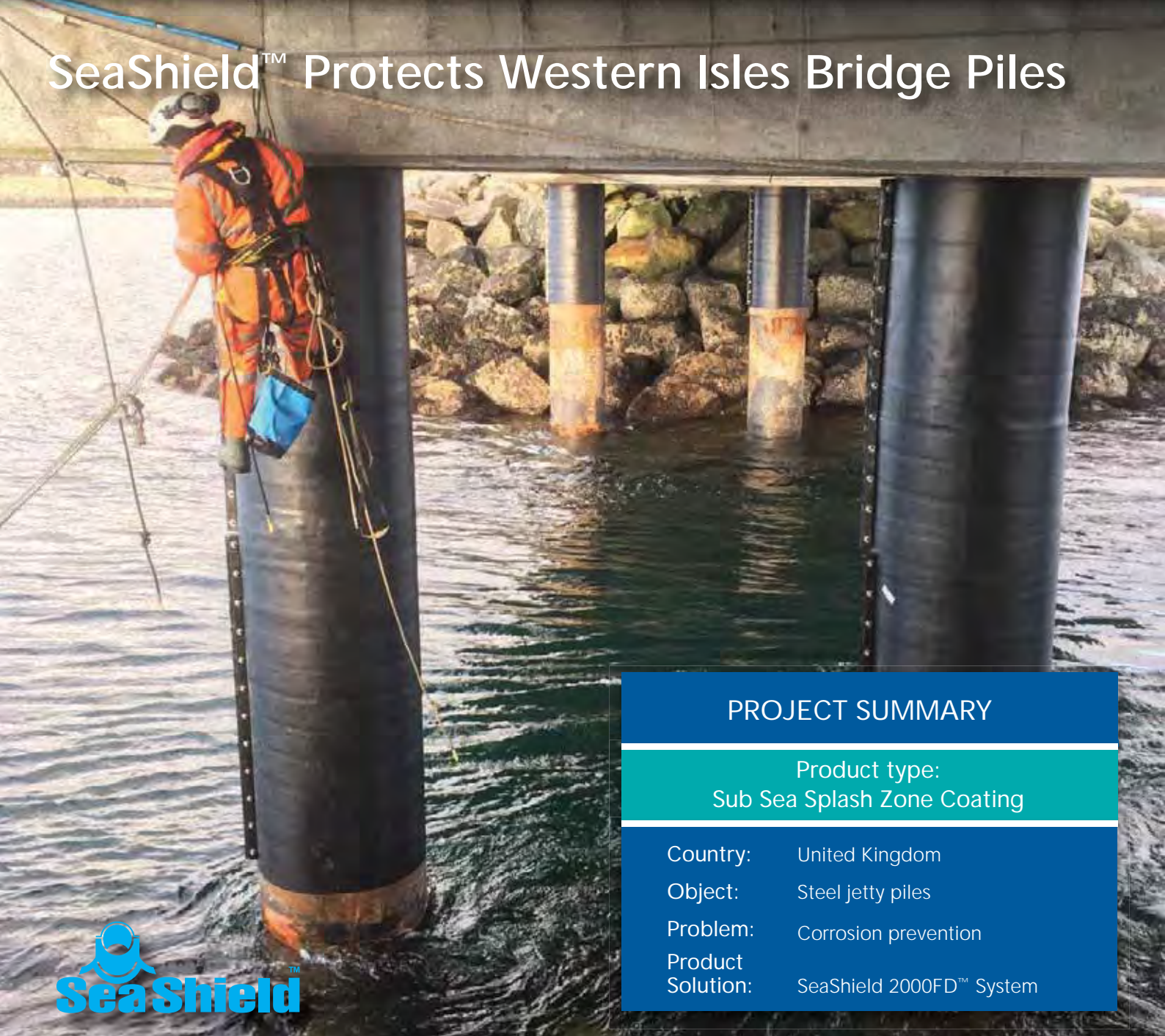
The completed application of the Seashield 2000FD™ System.
