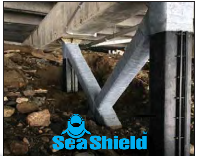
Below: Steel cross beams protected with Denso Glass Outerwrap 70™ in lieu of the 80 mil HDPE Outercovers.
