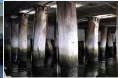
View of the timber piles beneath the Appleton Dock.
