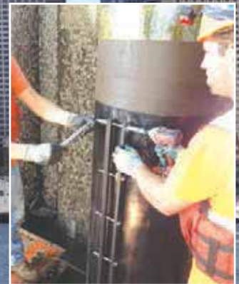
Installing the 80 mil HDPE outercover with M10 316SS fasteners
