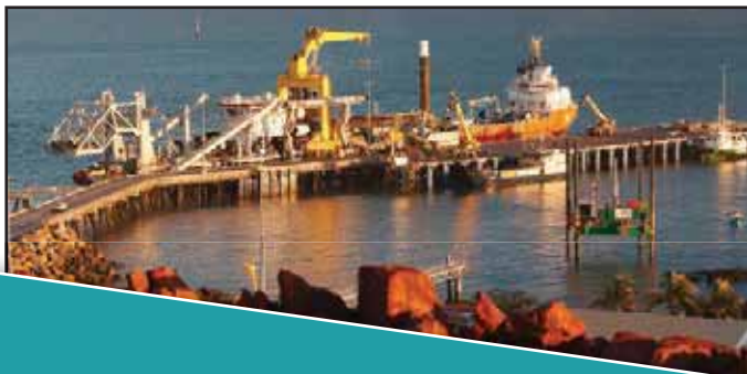
The busy MOF Wharf.
