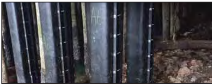
Completed H-Piles fully protected with the SeaShield Series 2000HD System.
