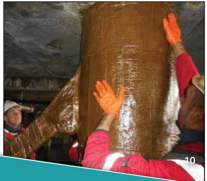
Wrapping the jetty piles and beams with Denso Marine Piling Tape.
