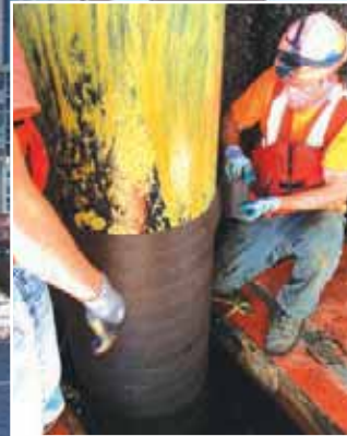
Installation of Denso S105 Paste™ and Densyl™ Tape to a 24" steel pile.
