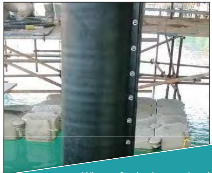
Below: The protective Jackets are applied completing the SeaShield 2000 FD system.
