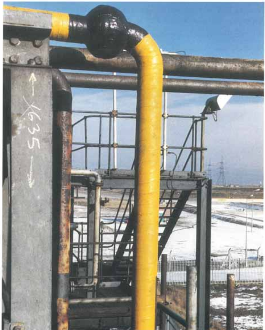
Close-up of pipe and flange showing completed Denso Covercoat System.
