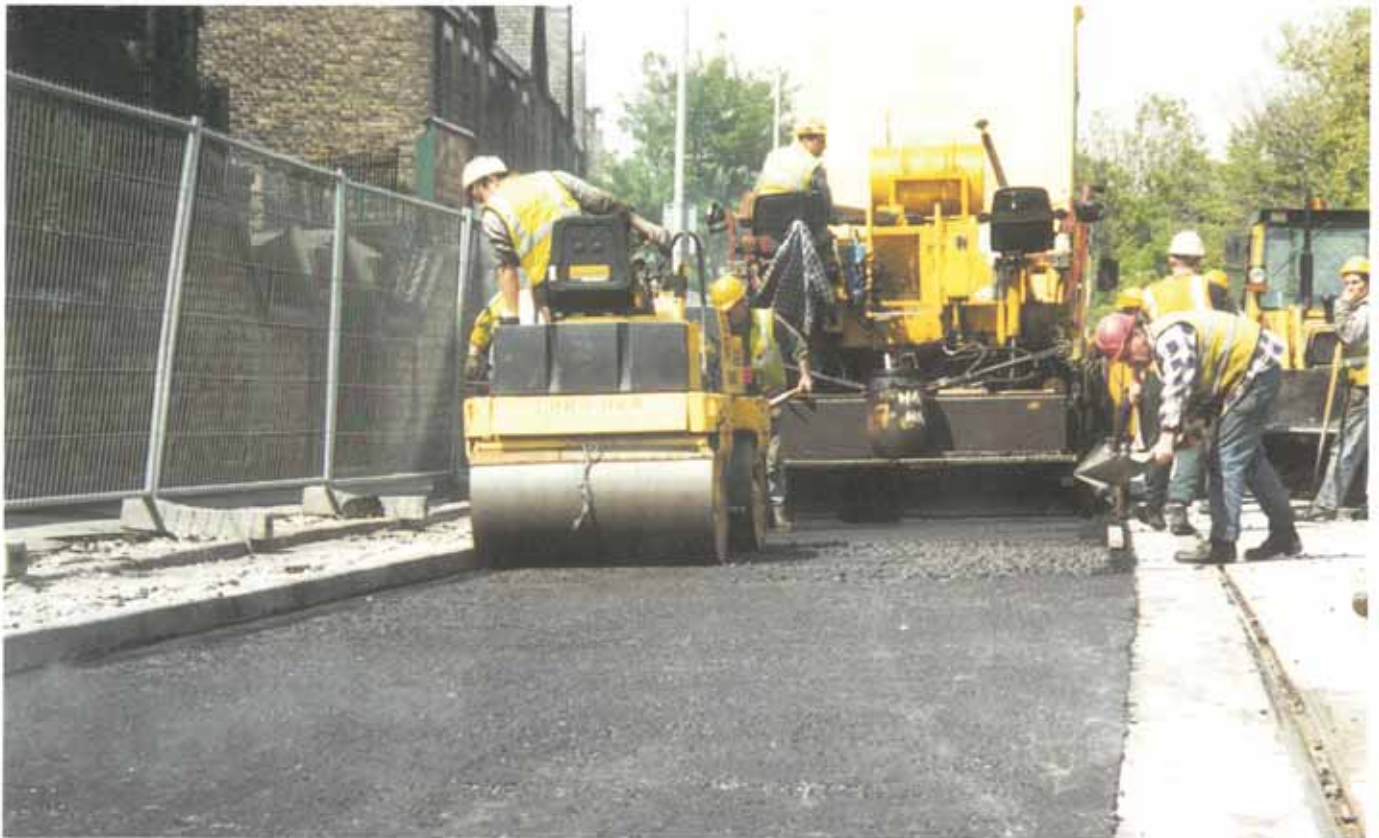
Rolling wearing course to complete carriageway modifications.
