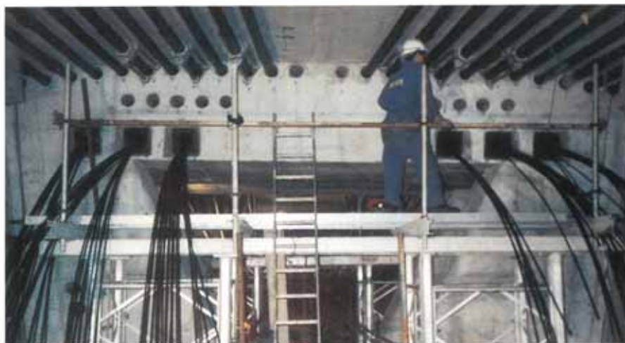
Insertion of cables into the ducts.
