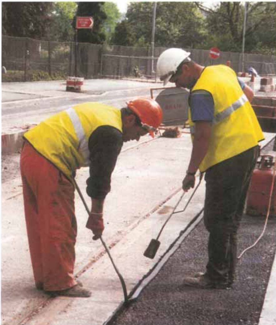
Application of Tokband Spezial to edge of concrete tram track bed.
