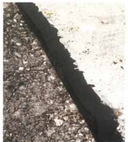
Close-up demonstrating the conformability of Tokband Spezial to the concrete joint face.
