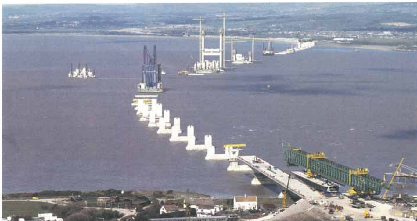
The Crossing during construction.
