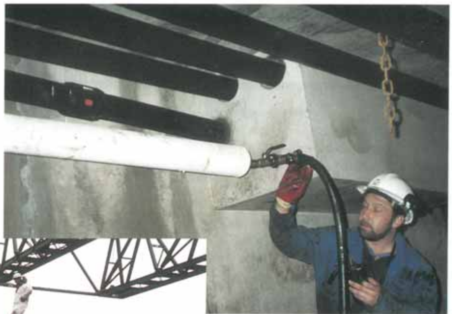
Pumping Denso Void Filler into the ducts.
