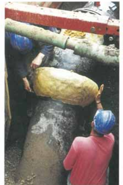
Smoothing joint contours with Denso Profiling Mastic.
