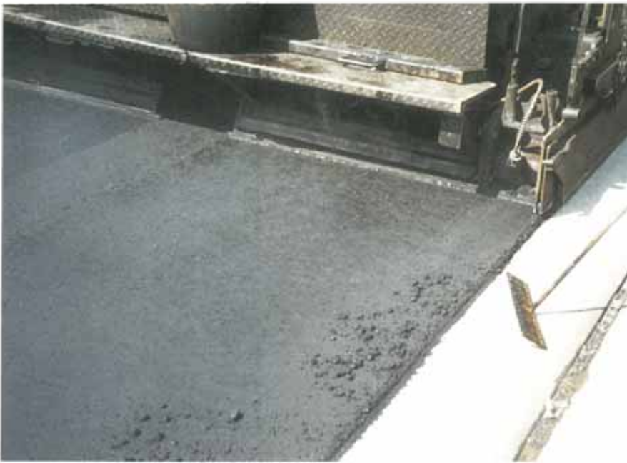
Laying asphalt wearing course against Tokband Spezial.
