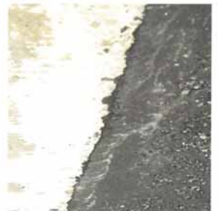
Close-up of completed flexible joint.
