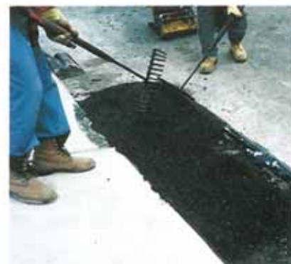
A flexible, waterproof bond between the new asphalt and the existing road surface is one of the main benefits of using Densoband.
