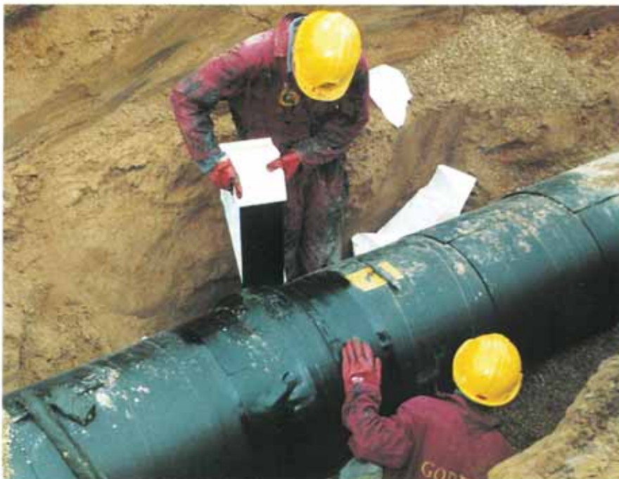
Densyl Mastic was used to smooth the contours of the joint before wrapping with tape.
