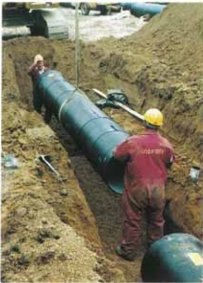
A pipelength being lowered into position.
