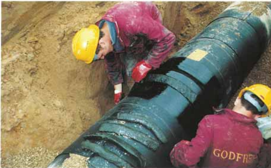
Densyl Mastic was used to smooth the contours of the joint before wrapping with tape.
