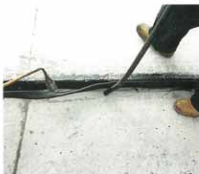
Densoband is hot applied to the vertical joint face.
