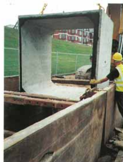
One of the box culvert sections is lowered into position.
