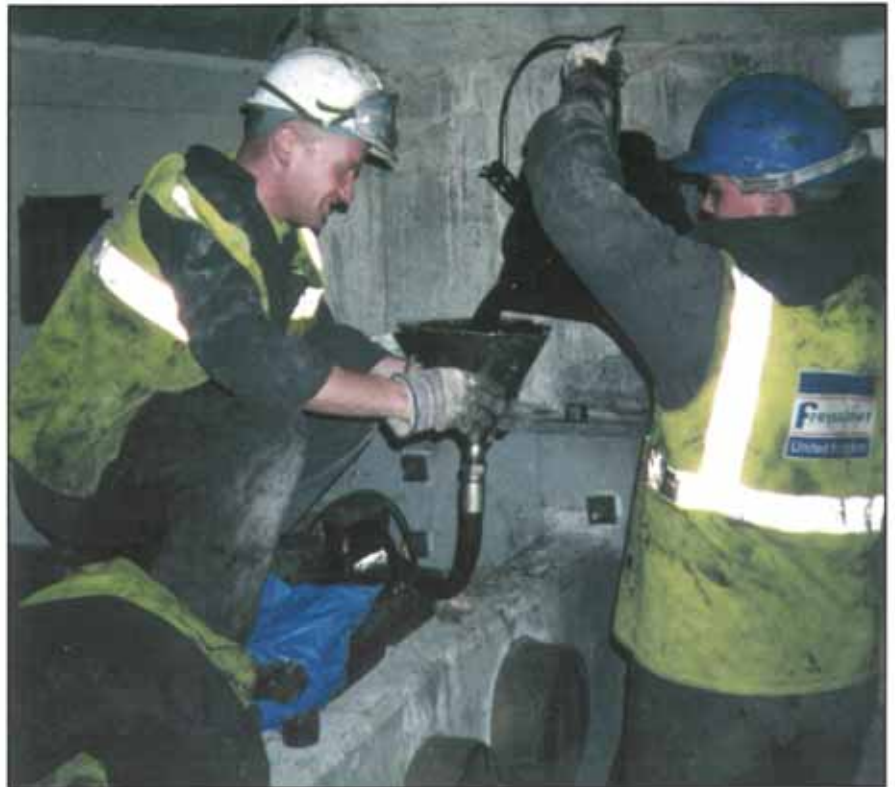
Application of Denso Void Filler to the prestressed cable end caps
