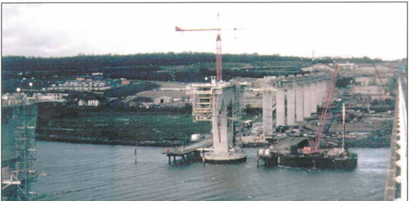
The Medway bridge under construction.
