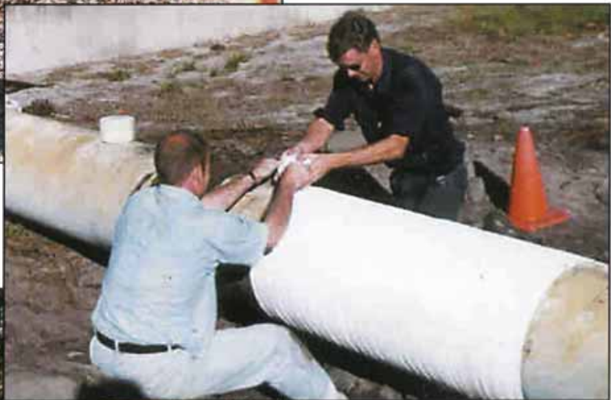
Centre: The Denso Steelcoat 300 System was exceptionally quick to apply.
