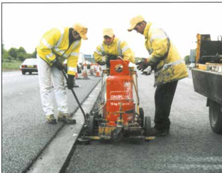
Above: Heating Densoband with a torch ensures an excellent bond with the vertical joint face. Below: The Densoband Applicator Machine was used for fast reliable application of the product.
