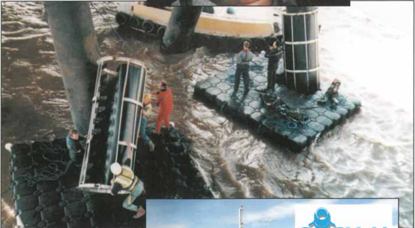
Below: Installation of the SeaShield Jackets using the special hinged cage devices.
