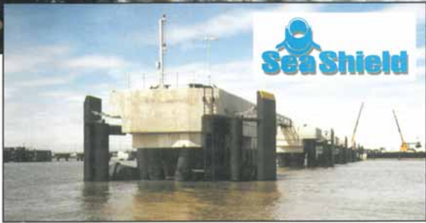
The Humber Sea Terminal Ro-Ro Berth.
