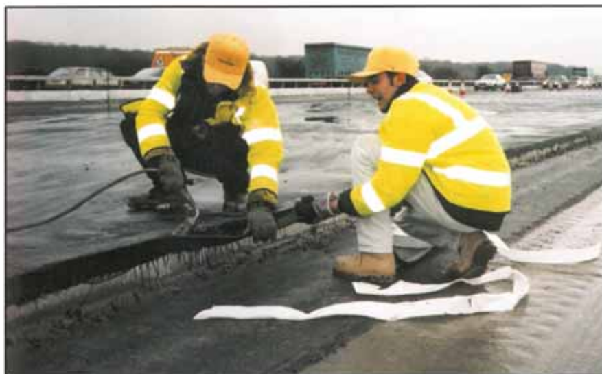
Above: Heating Densoband with a torch ensures an excellent bond with the vertical joint face. Below: The Densoband Applicator Machine was used for fast reliable application of the product.
