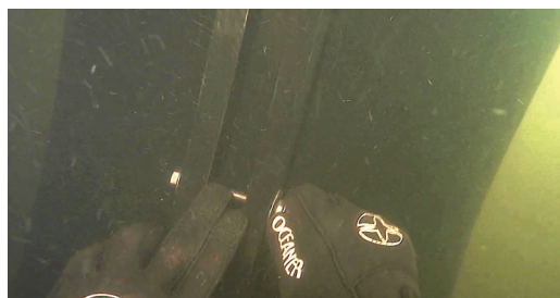
Installation of the HDPE outerjacket below water.
