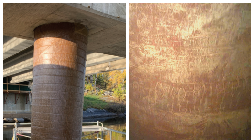
Installation of the Marine Piling Tape above and below water. Note the visibility of the spiral weld indicating a nice tight application of the tape.
