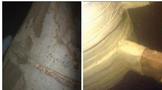
Cleaned steel pile below the waterline. Note the visible spiral weld. Installation of the LT tape and Glass Outerwrap at the structural cross-connection area.
