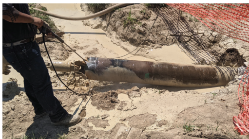
Pipeline with Denso Bore-Wrap® exiting drilled hole and being cleaned for inspection.
