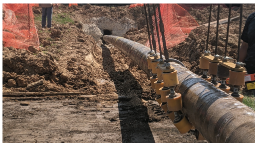
1,200 feet of pipe encapsulated in Denso Bore-Wrap® to protect the mainline coating prior to HDD installation.
