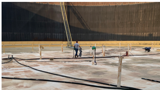
Sweep blasting over existing coating.
