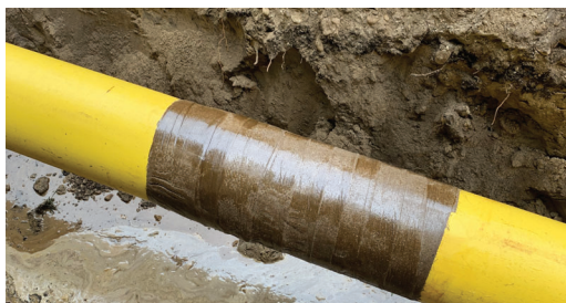
Bore-Wrap finished look with the seams fully fused together. The Contractor removed the Poly-Wrap as the pipe was being pulled.
