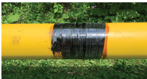
Typical weld joint on a 300 mm (12") yellow jacket steel gas main covered with bituminous tape for corrosion protection.
