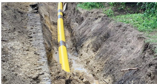
Image of the 300 mm (12") yellow jacket steel gas main in the process of being pulled.
