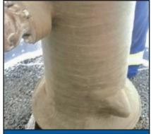
Phase 1: The application of Denso<sup>™</sup> LT Tape over the Denso<sup>™</sup> Paste.
