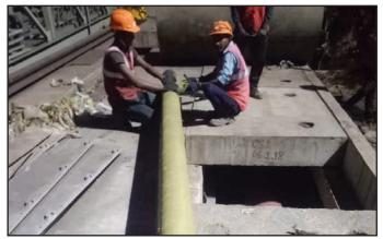
The prestressed cable sleeve is applied with Denso Paste™ before being spirally wrapped with Densyl™ Tape.
