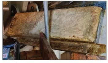
A wrap of Denso™ Hi-Tack Tape completes the Steelcoat 100 System.
