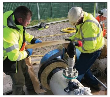
Above: Densoclad™ Tape is wrapped over Denso Profiling Mastic™ as part of the Denso P2 System™.
