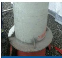
Phase 1: Spool piece cleaned and ready for the Denso<sup>™</sup> 'Above Grade' system.
