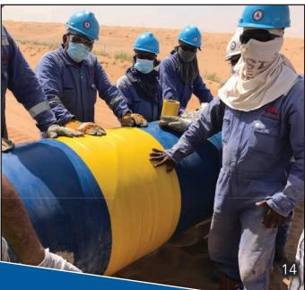
Denso<sup>™</sup> PVC Self-Adhesive Tape also applied with a 55% overlap.
