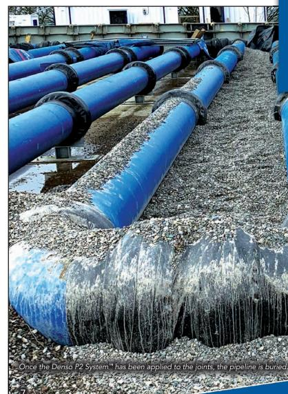
Winn & Coales recommended their Denso P2 System<sup>™</sup>, proven to effectively protect ferrous pipes, joints and fittings from the costly effects of corrosion. Fully compliant with the P2 Civil Engineering Specifications for the Water Industry (7th Edition), this time-proven system can be easily applied on-site before the pipe is buried – providing long-term corrosion prevention for the project at Pex Hill.
