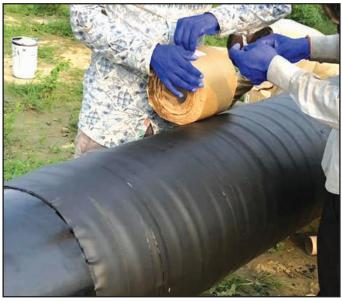
Densoclad 70HT<sup>™</sup> Tape is spirally wrapped around the pipeline.
