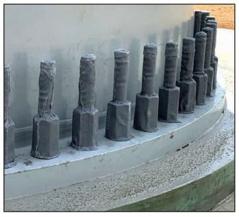
Denso  $^{\rm M}$  ColorTape recently installed on 76 exterior anchor bolts on wind turbine tower
