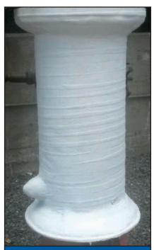
**Phase 1:** A coat of Archco<sup>™</sup> 15 Acrylic Topcoat completes the 1<sup>st</sup> Denso system.
