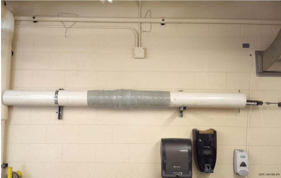
Figure 7. Wall-mounted pipe used for tension testing.
