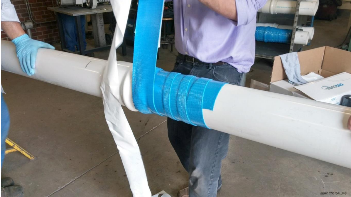
Figure 1. VISCOTAQ wrap being applied by Chuck Holt on June 2, 2015.
