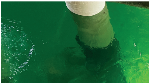
SeaShield Series 2000HD System being installed underwater.
