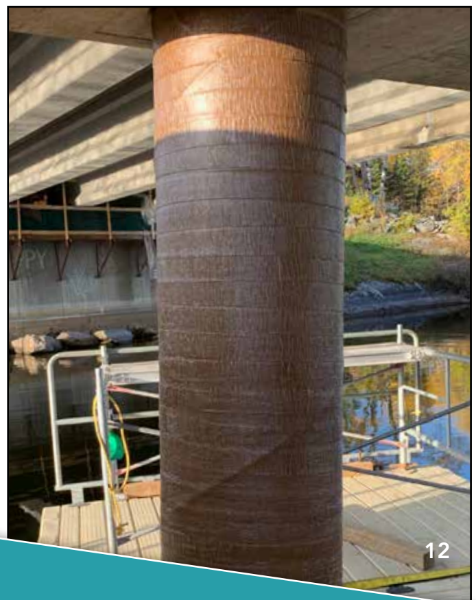
Marine Piling Tape is applied prior to 2000HD Jacket application.
