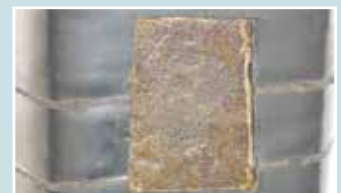
Outer layer panel removed to inspect the condition of pile surface.
