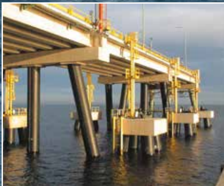
SeaShield System protecting jetty support piles - Libya.
