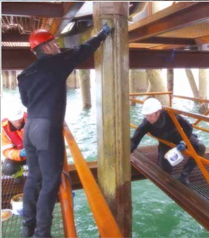
Applying the SeaShield Paste S105™ to a cleaned jetty pile.
