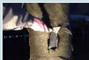
Marine Piling tape layer removed to check condition of pile surface.
