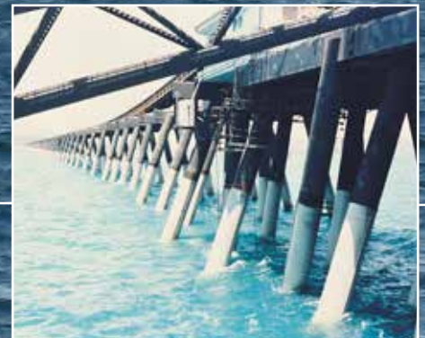
SeaShield System protecting coal loading jetty support piles - Australia.
