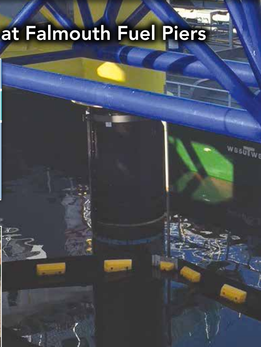
Above: SeaShield 2000FD™ protection for support piles on the new pier.
