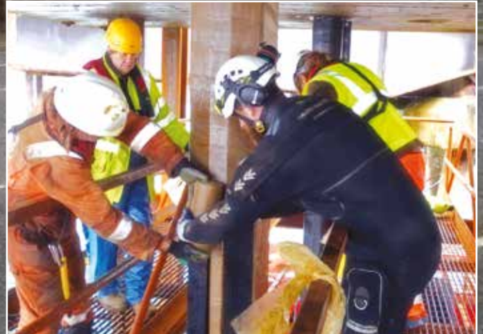
The application of SeaShield™ Marine Piling Tape.
