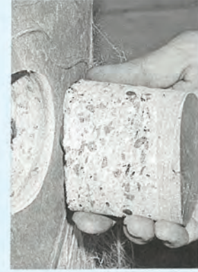
Core shows monolithic bond to concrete.
