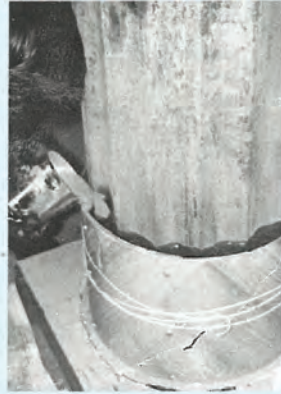
FX-70-6 Hydro-Ester mortar is poured through salt water solution.
