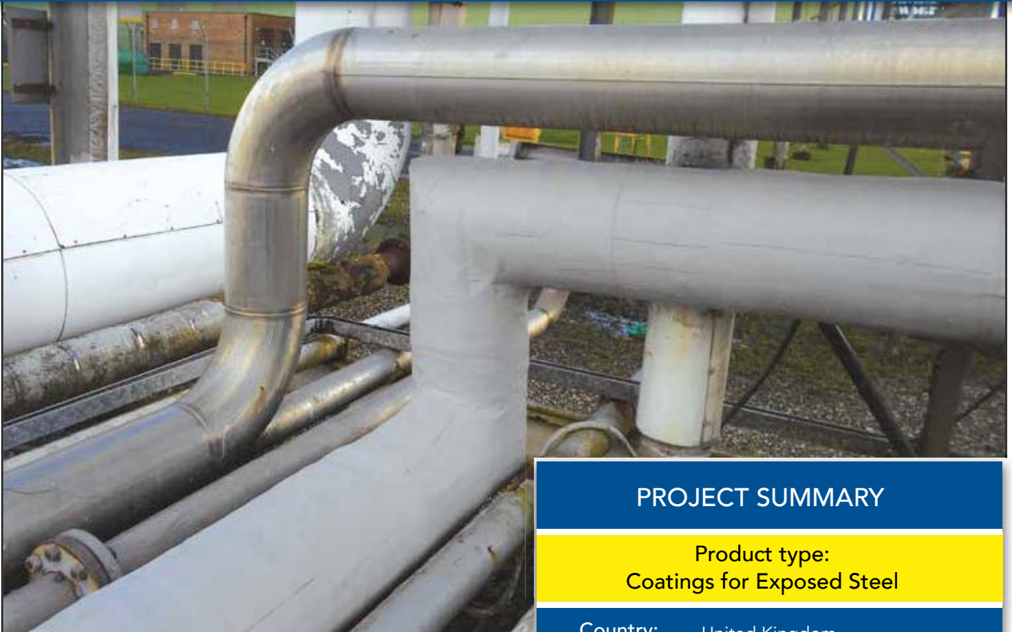
A coat of Denso Acrylic Topcoat completes the Steelcoat system.
