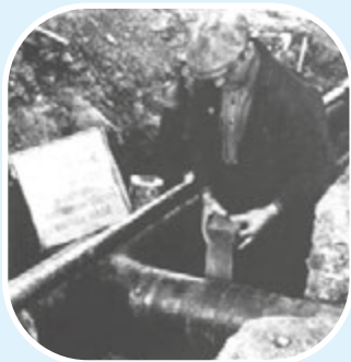
Early Densotherm and Denso Tape applications.
