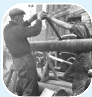
Early Densotherm and Denso Tape applications.
