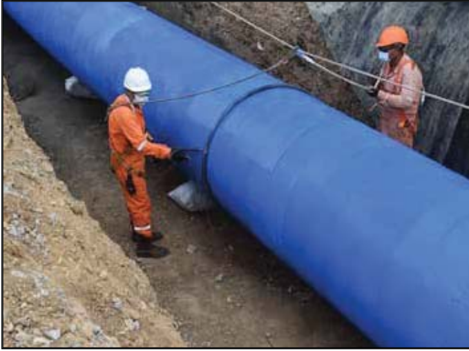
Holiday detection equipment used for routine check.
