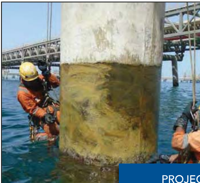
Above: After cleaning, the SeaShield Paste S105 is applied.
