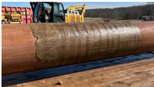
Bore-Wrap in 2 layers protects the anti-corrosion from damage.
