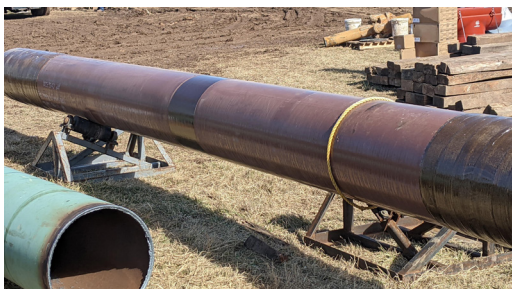
Test pull pipe with 3 options for protection.
