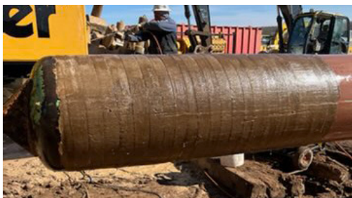
Pull-head after installation with 4 layers of Bore-Wrap.
