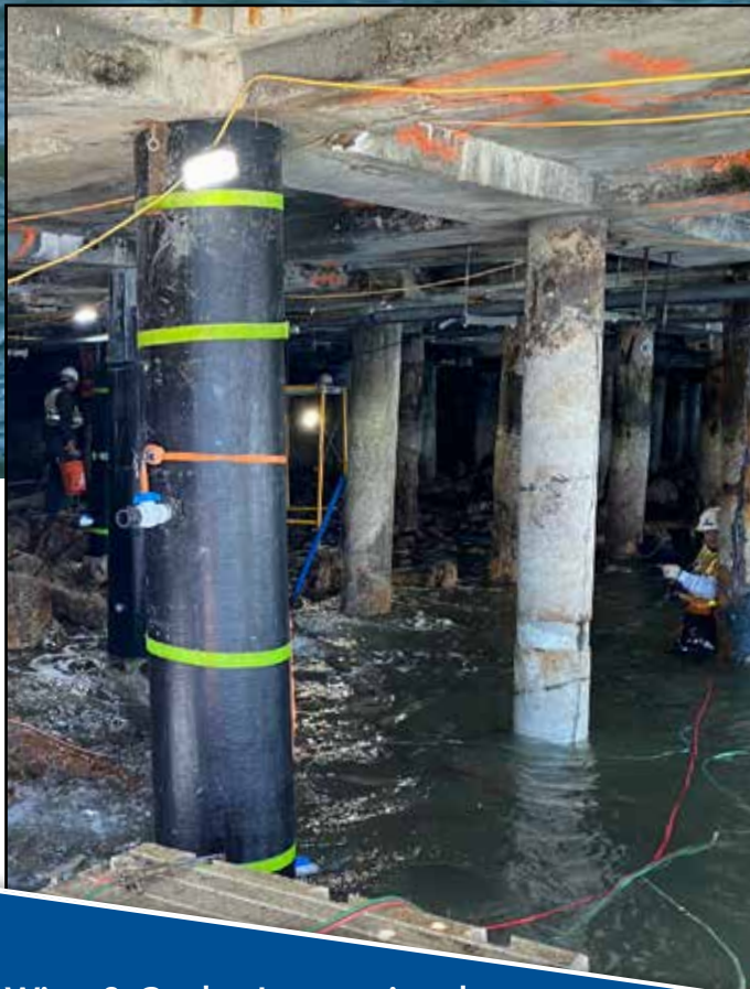
Below: The installation of the SeaShield™ systems underway.
