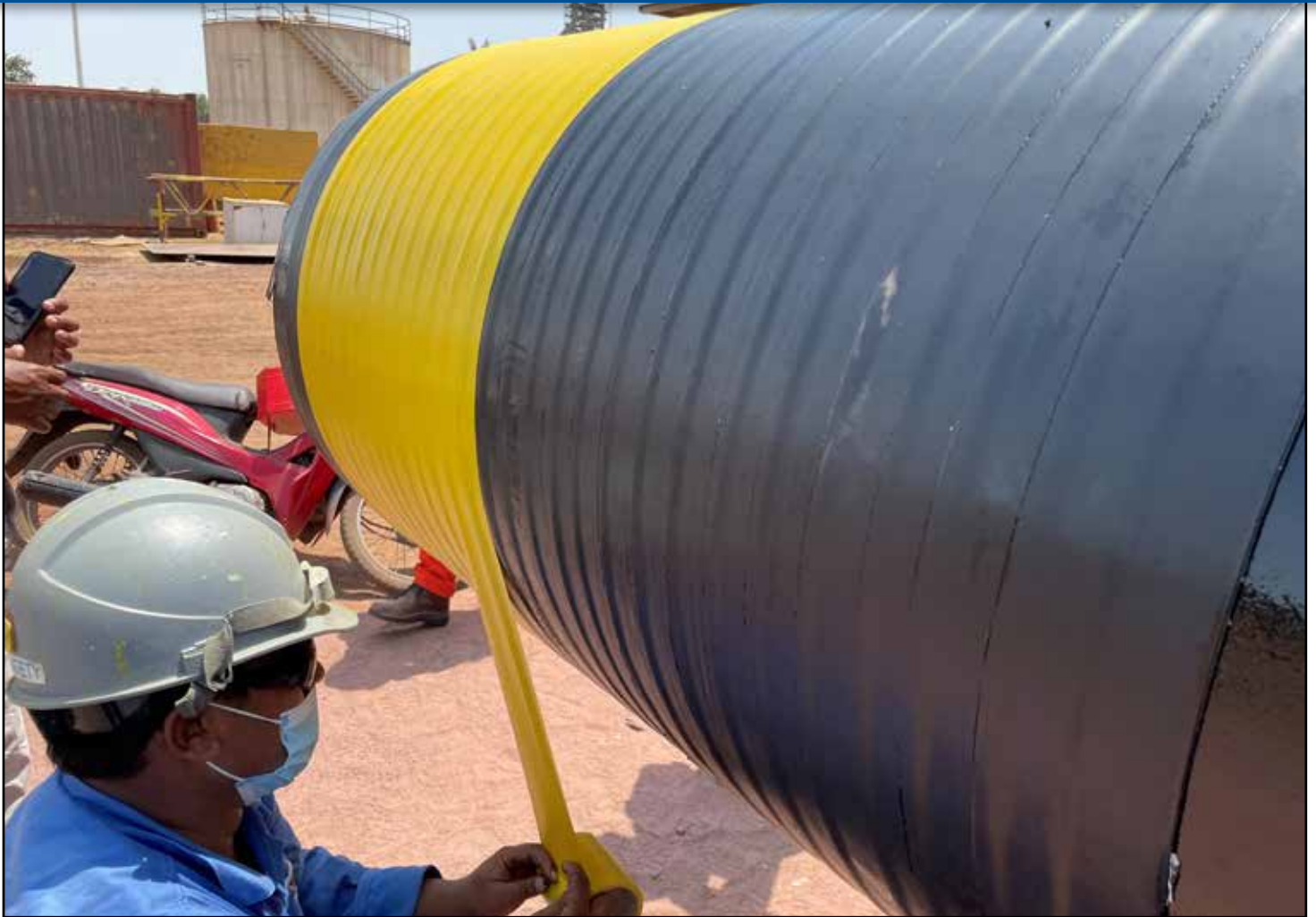
Denso PVC SA Tape™ is applied to the pipe lengths over the Densopol 80HT™, to give extra mechanical protection during transportation to the jobsite.
