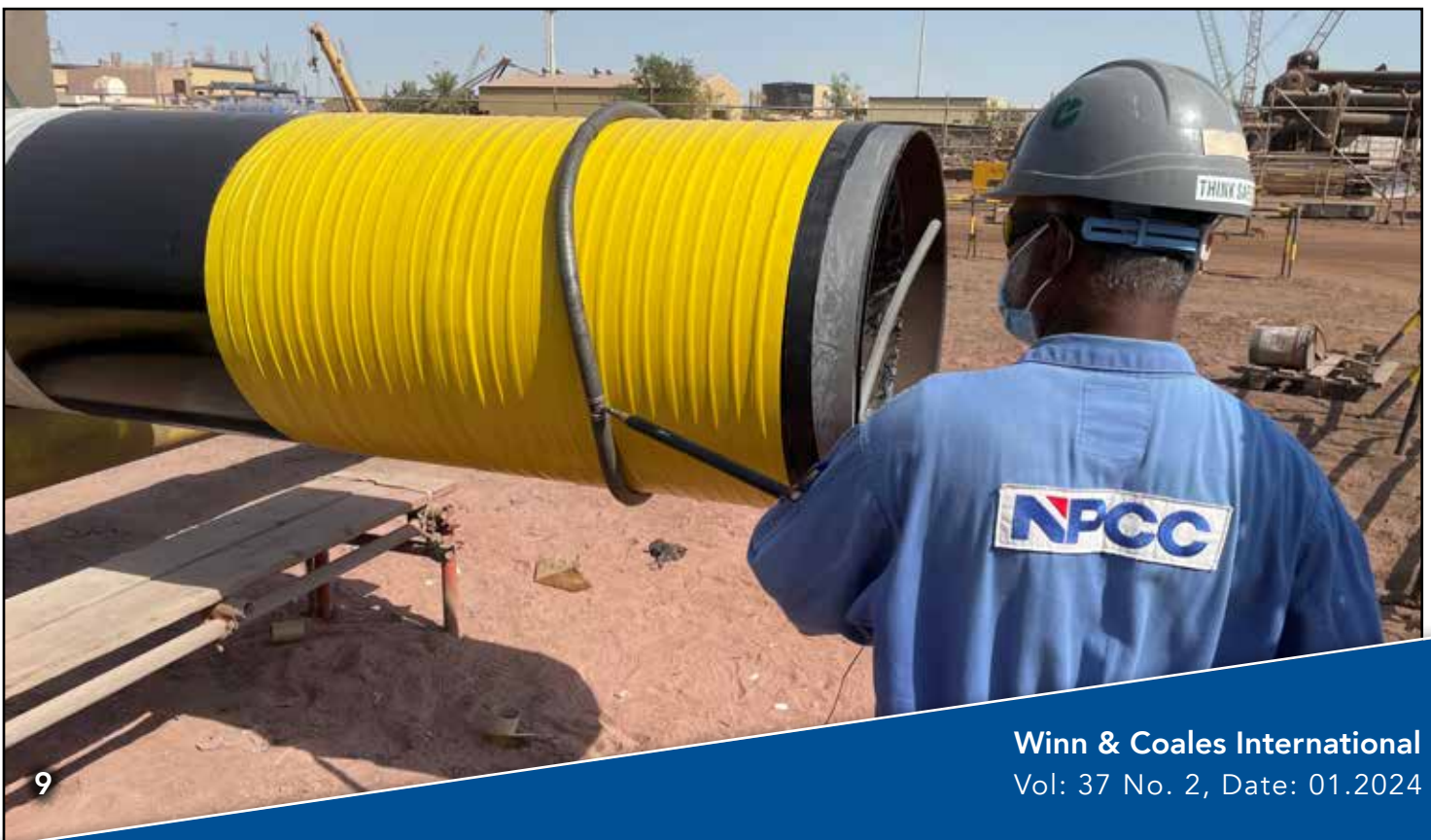
Denso PVC SA Tape™ is applied to the pipe lengths over the Densopol 80HT™, to give extra mechanical protection during transportation to the jobsite.
