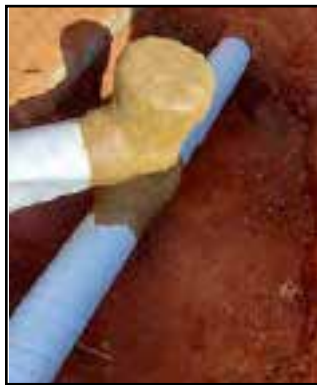
Denso™ Profiling Mastic and Denso™ Butyl Tape System applied to the prepared areas.
