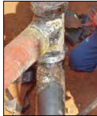
The surface condition once the existing shop applied coating was removed.
