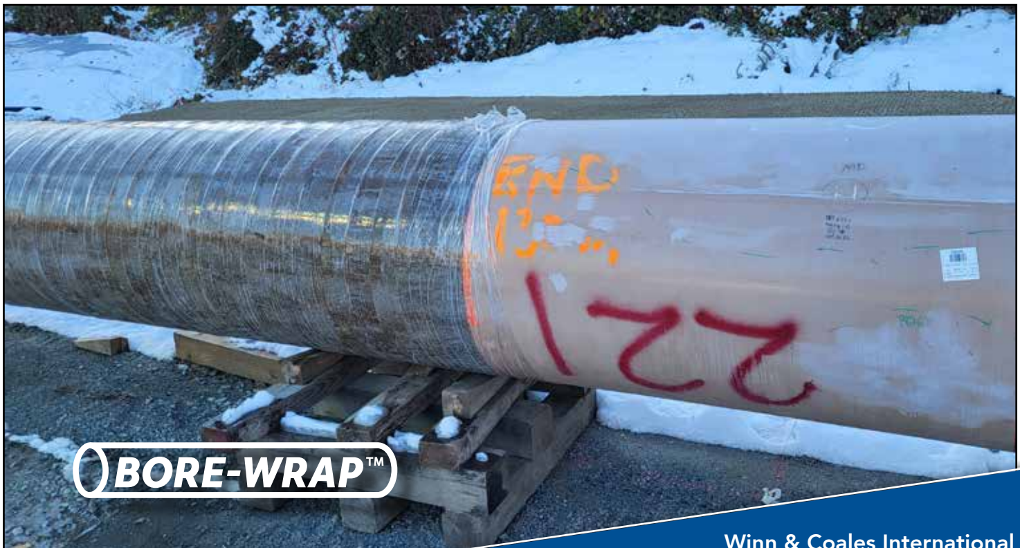
Denso Bore-Wrap™ application to wastewater pipeline
