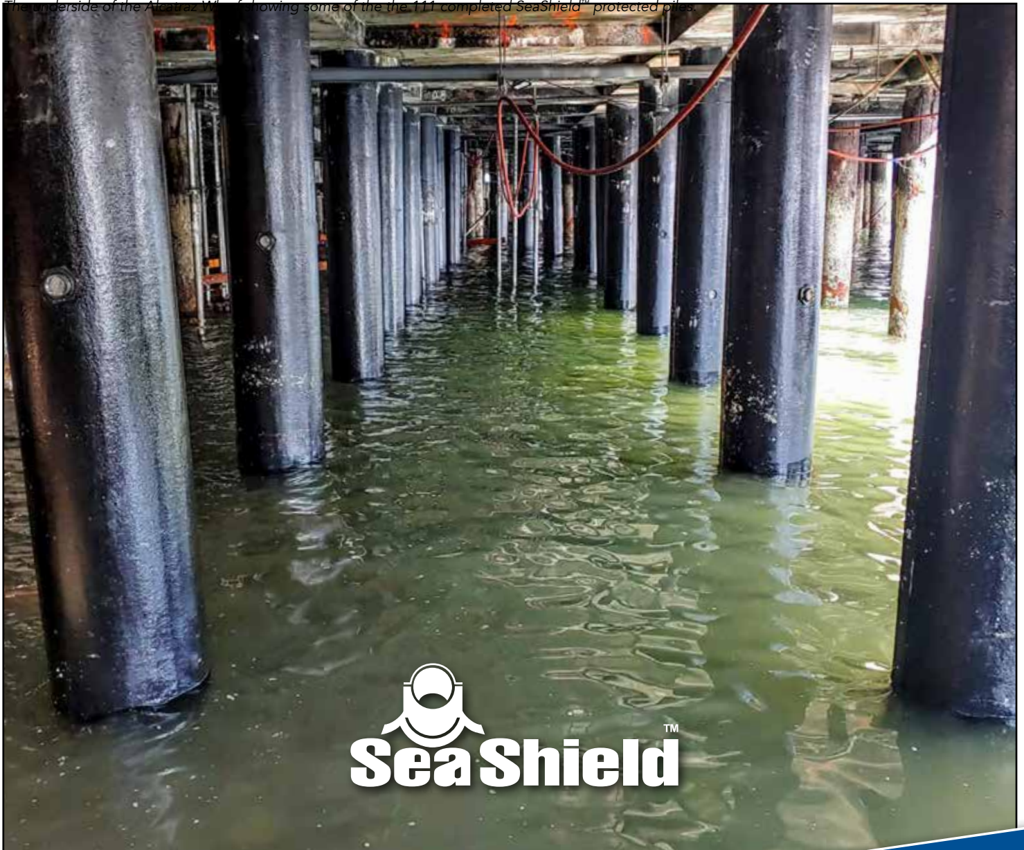
The underside of the Alcatraz Wharf showing some of the the 111 completed SeaShield™ protected piles.
