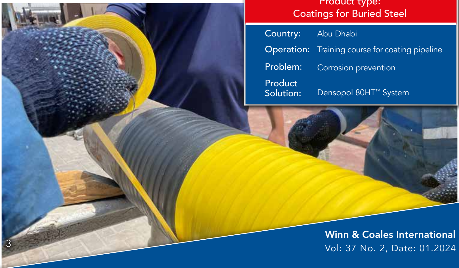
Below: Denso PVC SA Tape™ is then applied to the pipe lengths over the DensoPol 80HT™ for extra mechanical protection during transportation.
