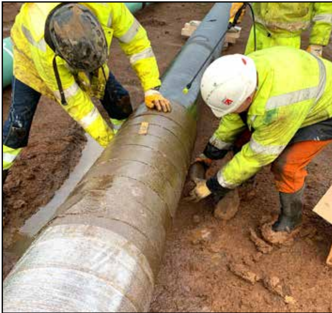
Denso Bore-Wrap™ is applied spirally with a 55% overlap to the pipe, followed by the application of Denso Polywrap™ to aid curing of the Bore-Wrap™.
