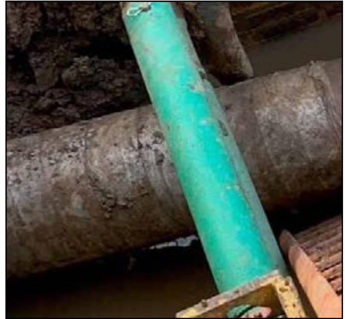
View of pipe after it had been pulled under the roadway. Denso Bore-Wrap™ is still intact so there is no damage to the pipe coating.
