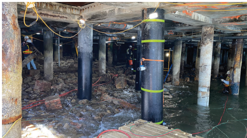
The installation of the SeaShield™ systems underway.
