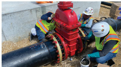
Denso Paste is easily applied to the substrate by gloved hand or brush as the initial application step.
