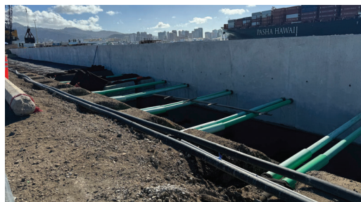
Protected with PVC piping before final burial.
