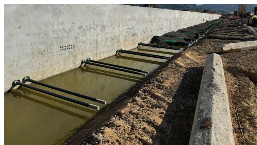
The Denso and Viscotaq tape wrap system installed on tie-bars.
