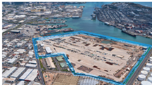
Kapalama Container Terminal Phase 2 during construction in late 2022.
