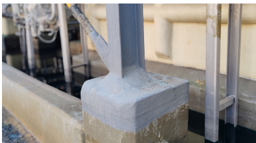
Completed Denso Covercoat System applied for column base protection.
