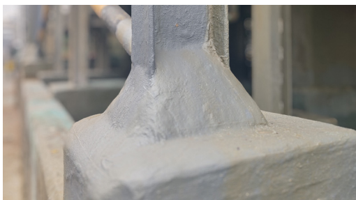
Full column base encasement system installed with Archco 15 flexible topcoat.
