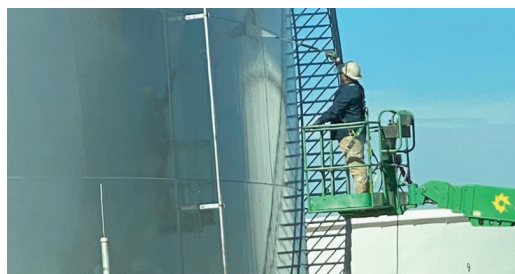
Pressure washing existing coating.
