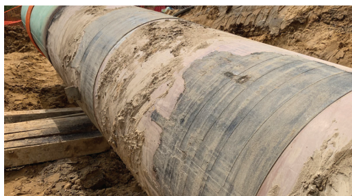
The Denso Bore-Wrap at the leading edge is still in place 360° around the pipe.
