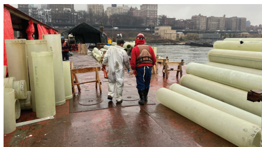
SeaShield Fiber-Form Jackets staged on barge.
