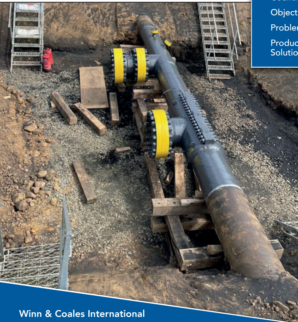
Wide angle view of the completed Protal 7300 (UK) application to the gas pipe in Dalmeny.
