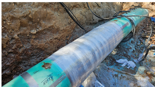
Completed section of the Protal 2800CF pipeline repair system in place.
