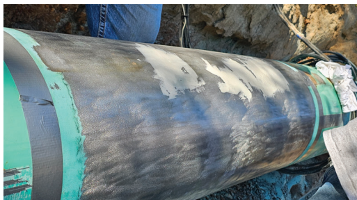
Protal 3210 Load Transfer Filler was applied.
