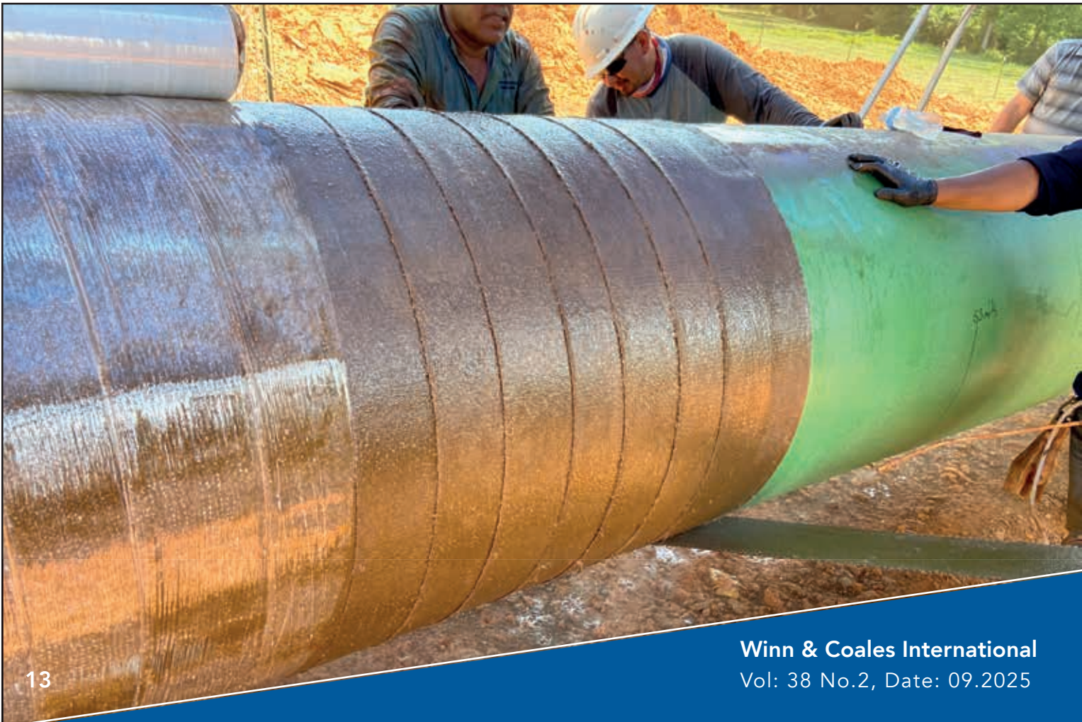
Below: Application of the Denso Bore-Wrap System
