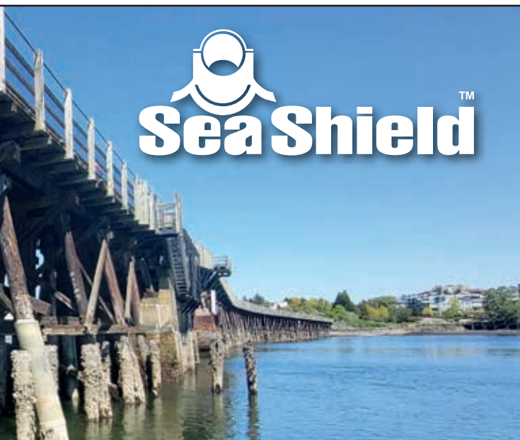
The completed SeaShield Series 400 System installed on the repaired piles.
