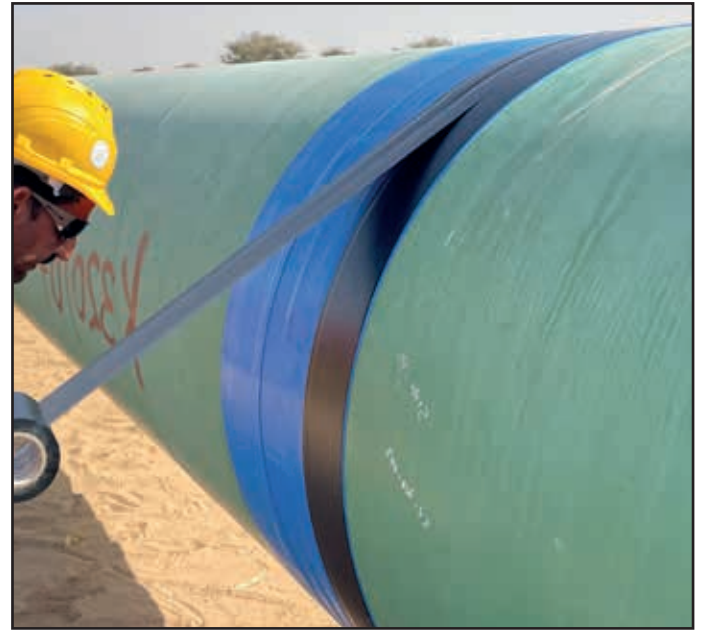
Application of the Viscotaq PVC Outerwrap.
