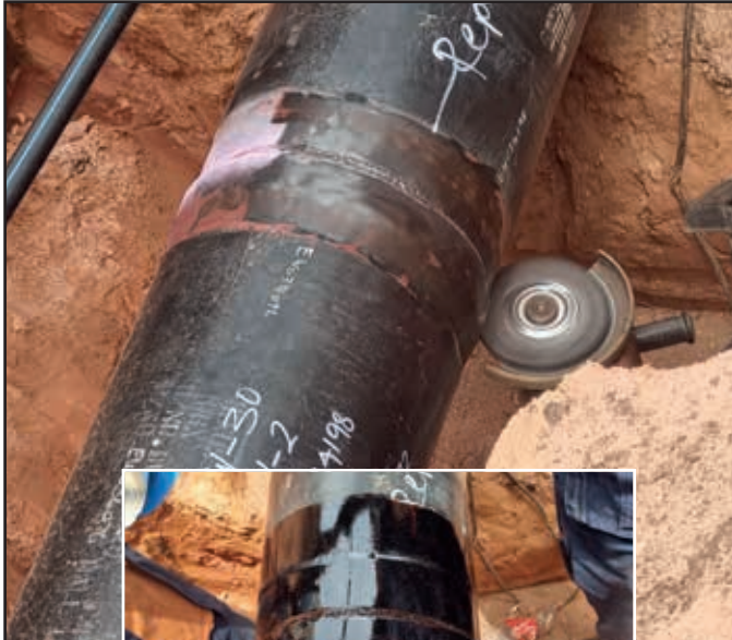
Preparation of the welded joint surface, using a hand-held power tool.
