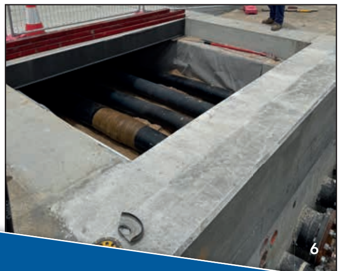
Below: View of buried pipelines post-application.
