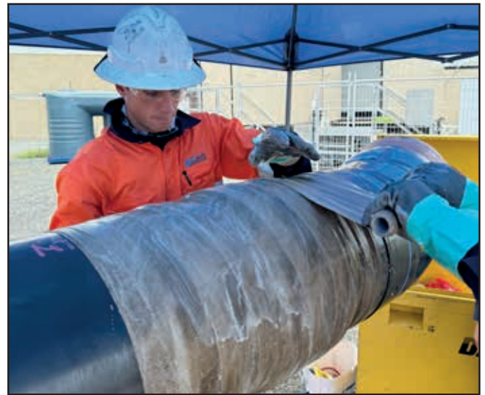
Above: Application of Denso™ Glass Outerwrap.
