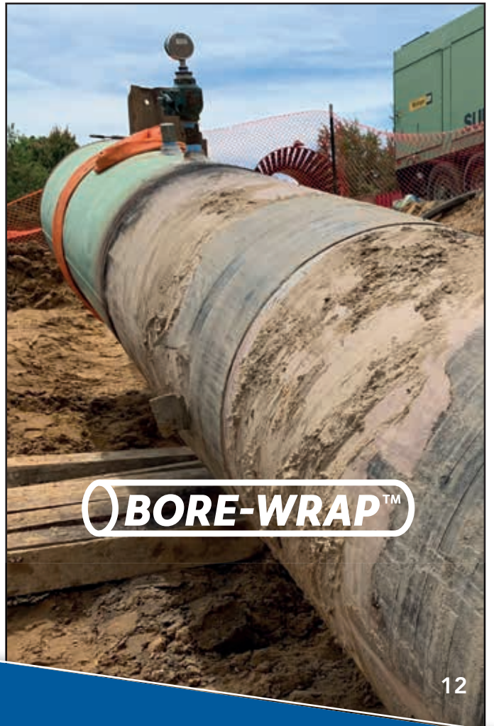
Above: The Denso Bore-Wrap™ is fully intact on the left after the pull.
