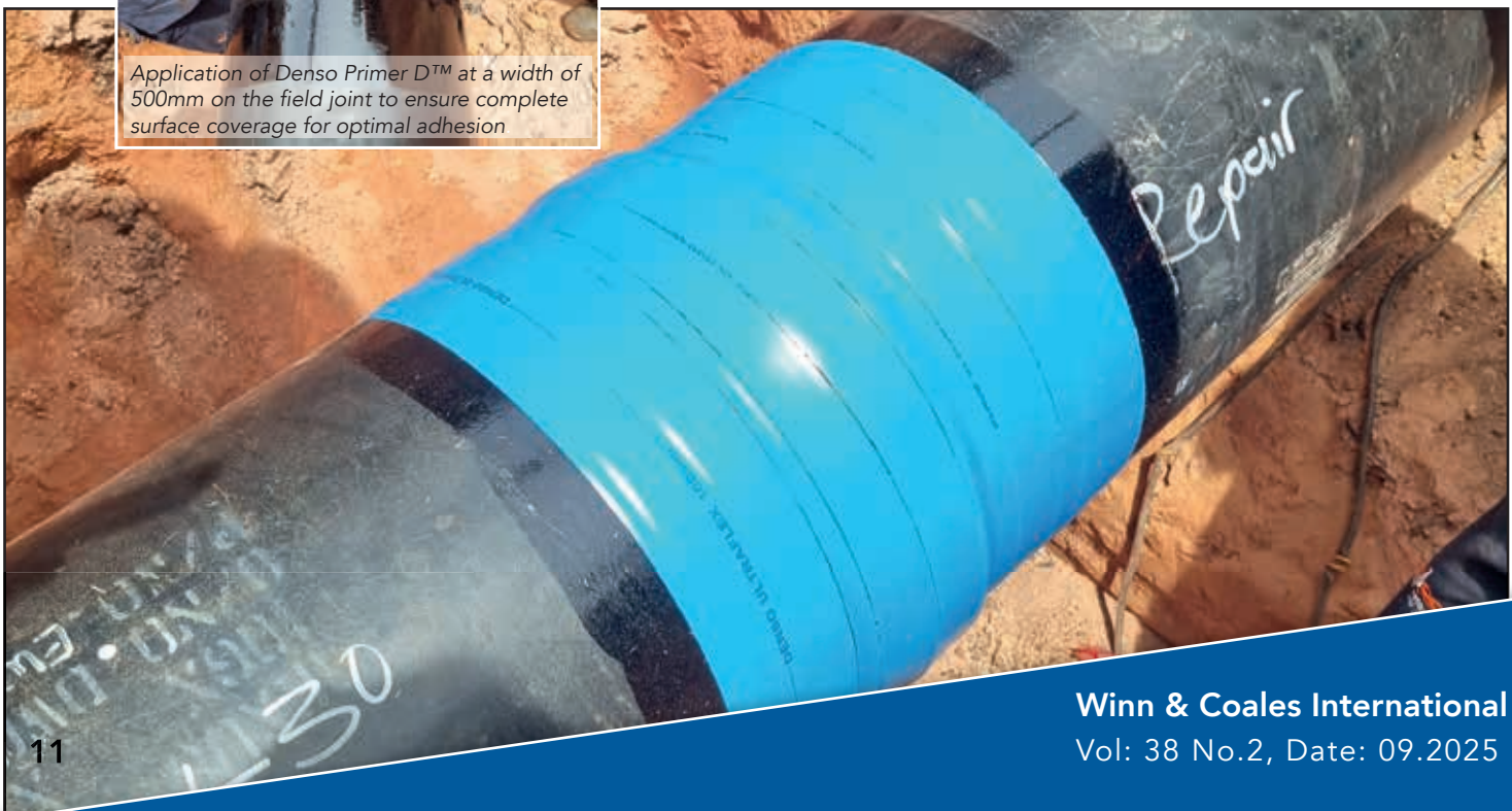
Below: The completed Denso welded joint protection.
