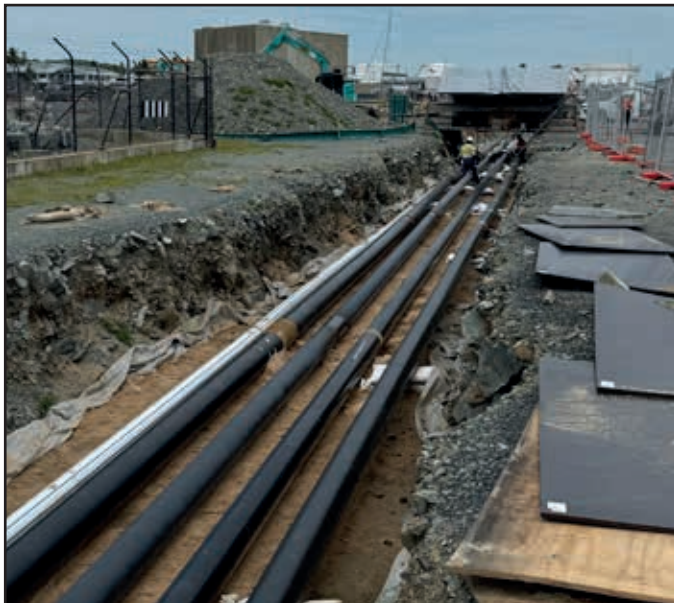
Above: Alternate view of the pipelines, post-application.
