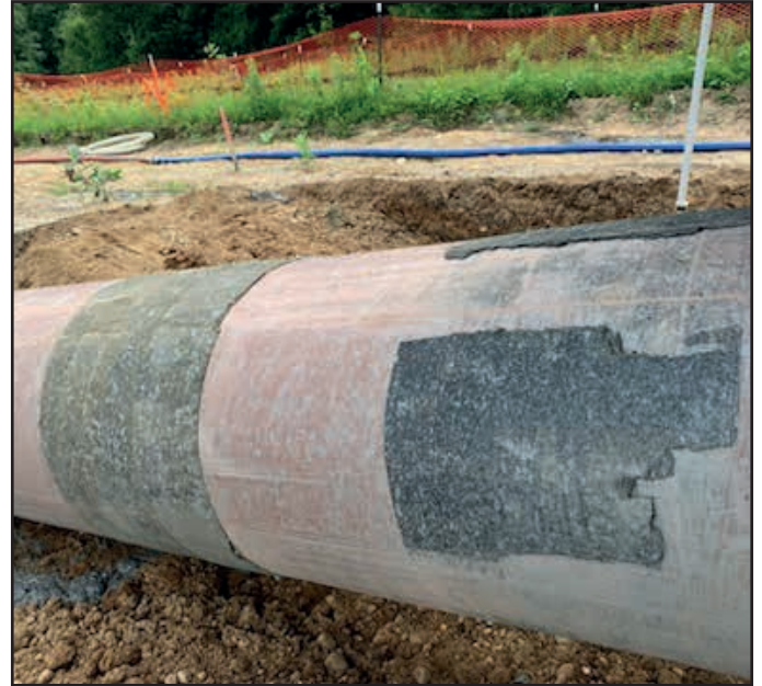
Above: The Denso Bore-Wrap™ is fully intact on the left after the pull.
