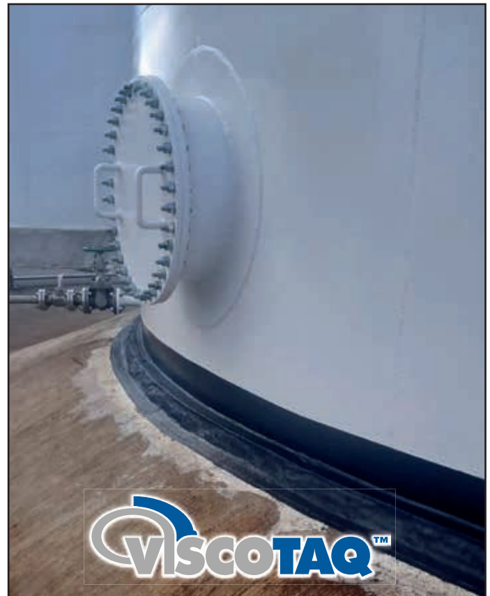
The Viscotaq™ Chime Sealing System applied to the fuel storage tank.
