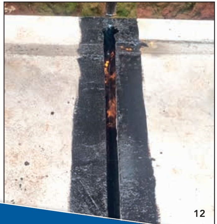
Denso Primer D™ & Denso™ Joint Sealer applied for all new concrete bases placed forward (external section).
