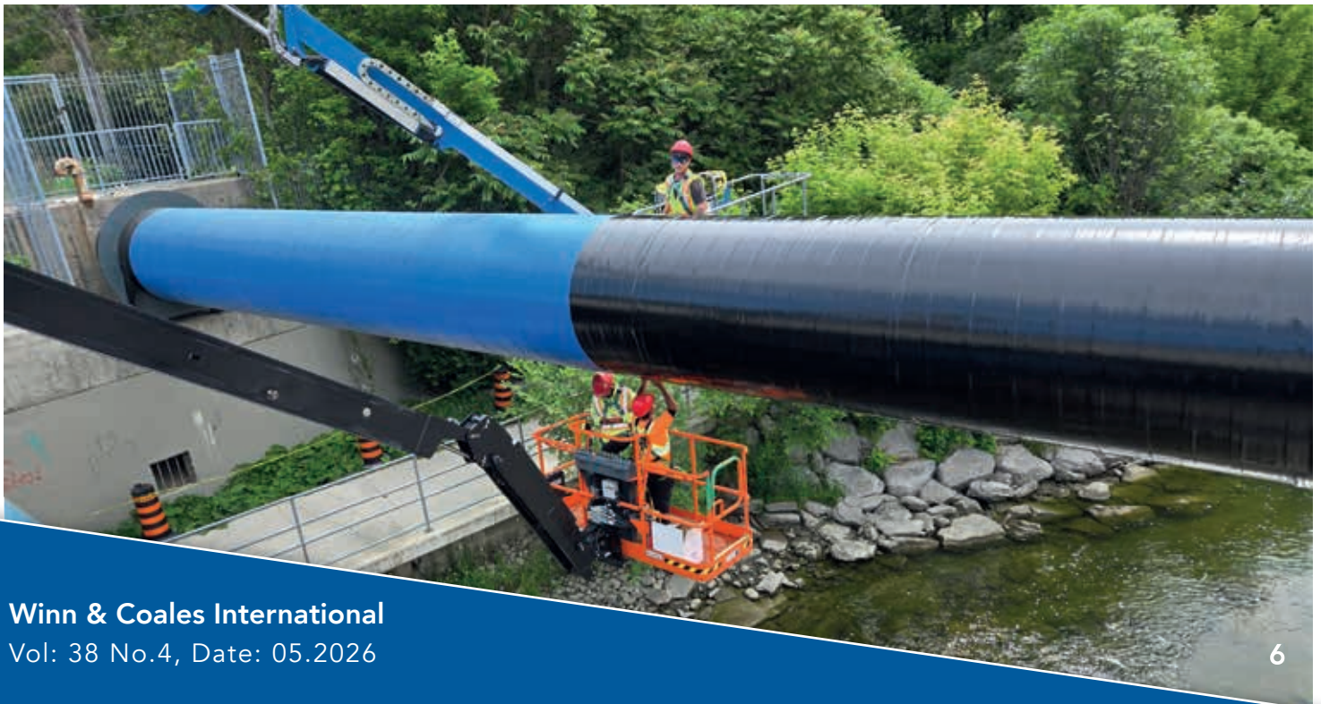
Below and top of page 9: A wrap of ViscoWrap™ ST (blue) is followed by a wrap of ViscoWrap™ PE (black).
