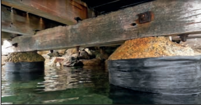
The completed SeaShield 70™ System.
