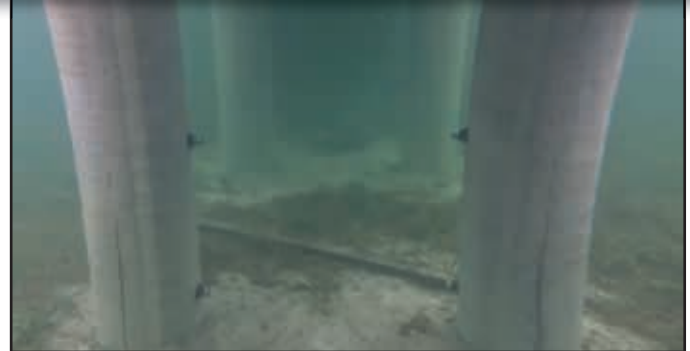
Underwater view of the completed SeaShield 400™ System.
