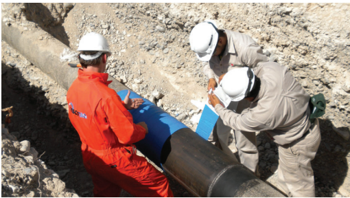
The Viscotaq system was easily installed over difficult pipeline legacy coatings with SP2 surface preparation.
