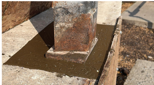
Structural silo foundation repair utilizing Denso 190DP Epoxy Grout.
