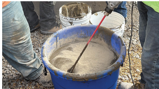
Denso 190DP Epoxy Grout is a high strength, low exotherm deep pour grout.
