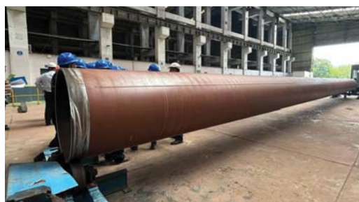
Full-length HDD pipe prepared for factory-line mechanical protection.
